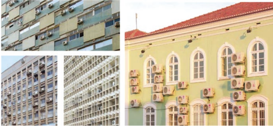
Fig. 3.147 Luanda, Angola: the use of air conditioning can be avoided through a correct use of passive design, reducing damage to the environment and operation costs
