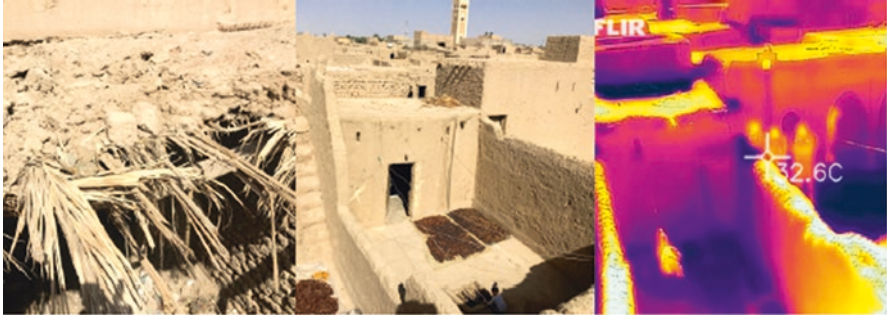
Figs. 3.128, 3.129 and 3.130 Morocco – on the left, example of floor slab (in ruin), allowing to understand its construction; on the centre, example of building construction in overlapping floors; on the right, thermal image of buildings' rooftops, clearly noticing the increased temperature on the roof slab and the progressive cooling of the elements on the lower floors
