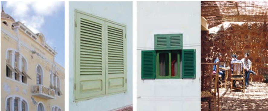
Fig. 3.34 Adjustable external shading: wood shutters (venetian blinds) provide shade and simultaneously allow for natural lighting and ventilation. (Right) Adjustable shading: leisure area in the fort museum, at the Cidade Velha. The shading strategy allows natural lighting and ventilation
