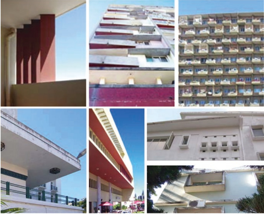
Fig. 3.40 Fixed shading in modern buildings, Maputo, Mozambique
