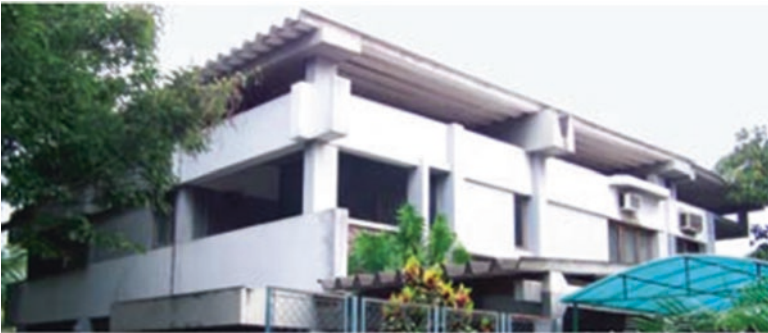
Fig. 3.78 Ventiladed roof, Maputo, Mozambique
