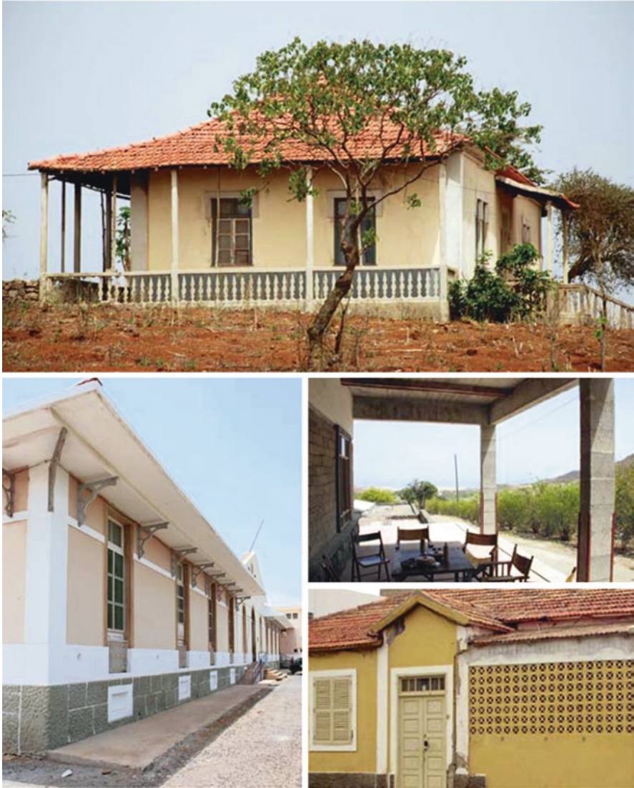
Fig. 3.32 Examples of fixed shading in Cape Verde: (1) projection of the roof to shade the facades, in the Amilcar Cabral house museum; (2) projection of the roof in institutional building; (3) shading of esplanade in Santo Antão; (4) grid system for shading and ventilation in a building in Mindelo; (5) vertical shading in a services' building in Praia
