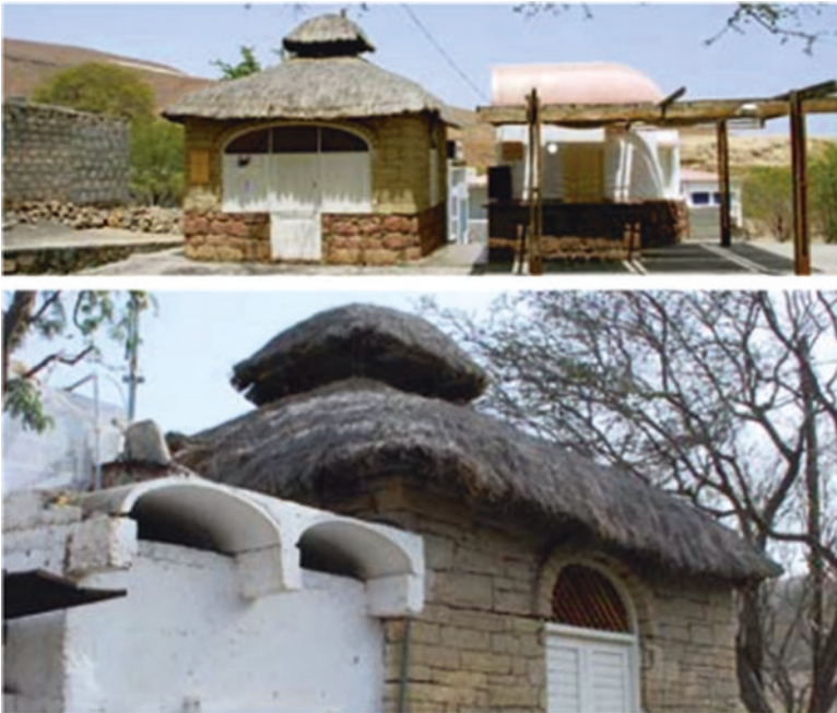
Fig. 3.104 Tourist information building in Santo Antão, using hollow concrete slabs and openings on the roof for ventilation
