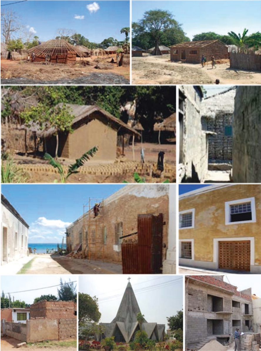
Fig. 3.110 In Mozambique, the use of massive building materials, like earth, stone, bricks or concrete, can be observed throughout the country. Above: adobe and stone vernacular houses in Ilha de Moçambique. Below: brick and concrete construction in Maputo (Tables 3.10 and 3.11)
