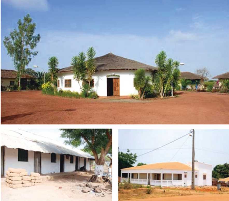
Fig. 3.51 Buildings painted white, in Guinea-Bissau, to reduce the discomfort from overheating
