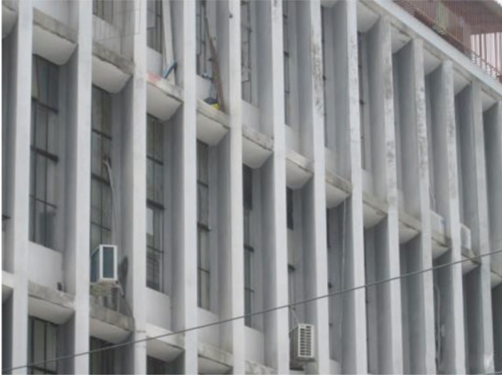
Fig. 6.16 Office building on East Timor Street
