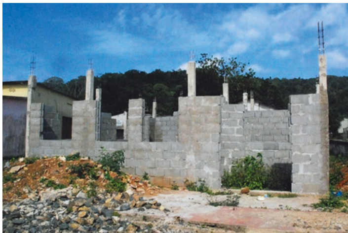
Fig. 13.8 Construction of a building with concrete blocks in S. Tomé island
