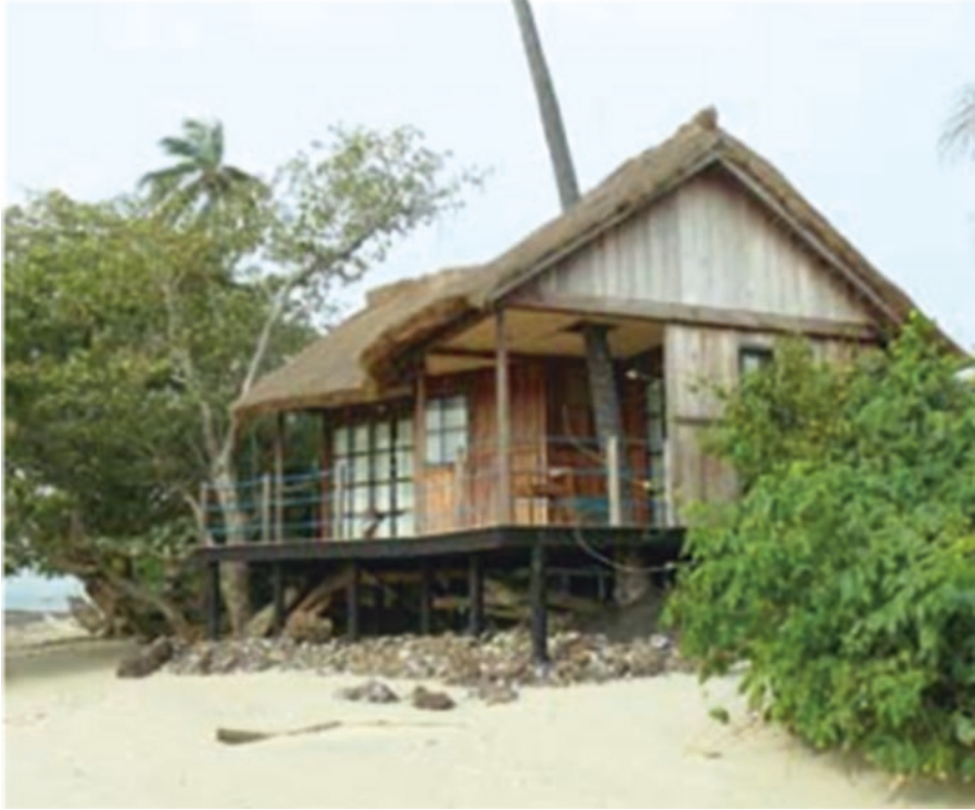
Fig. 3.109 Guinea-Bissau: the use of lightweight buildings may offer advantages in zones with low thermal amplitudes (below 8 °C between night and day during most of the year), where thermal inertia has little effect. Building features like elevated structures, ventilated roofs and wind-catching verandas can be used to improve ventilation
