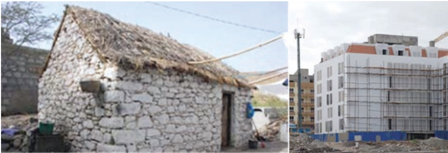
Fig. 3.48 Heat protection: (1) whitewashed vernacular house, on Santo Antão, (2) contemporary building painted white, in Mindelo, Cape Verde
