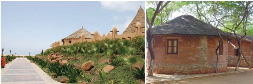
Fig. 3.54 Contemporary use of thatch: Hotel in Sal, Cape Verde (left), and Barra do Cuanza (Angola). Using this typology of local tradition also brings benefits of solar protection
