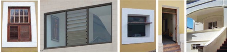
Fig. 3.70 Maputo, Mozambique: adjustable devices for natural ventilation
