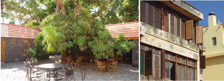
Fig. 3.26 Shading using vegetation in Cidade Velha (left). Adjustable wooden venetian blinds in modern building in Bissau (Guinea)
