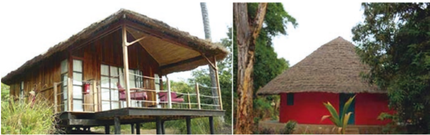
Fig. 3.4 Eco-tourism resorts in Bijagós (Guinea-Bissau): contemporary architecture inspired on local vernacular, with a good bioclimatic performance and use of local building materials
