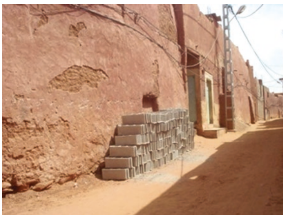
Fig. 4.26 Cement blocks as trusted building material
