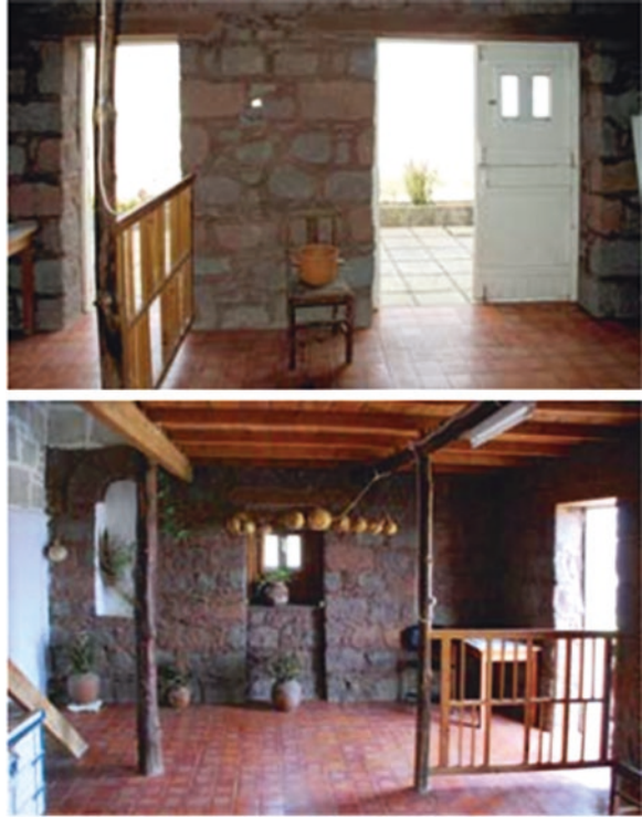
Fig. 3.63 Rehabilitated vernacular house in Santo Antão. The window area is sufficient and adequate to meet the needs of natural lighting and ventilation
