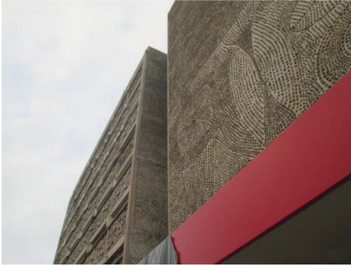
Fig. 6.26 Abreu, Santos e Rocha building
