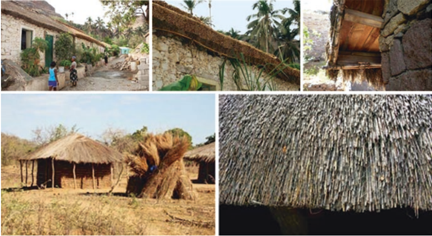
Fig. 3.53 Vernacular houses in Praia, Cape Verde (above), and Pemba, Mozambique (below), with thatched roofs. Thatch is an insulating material that protects the building against heat gains
