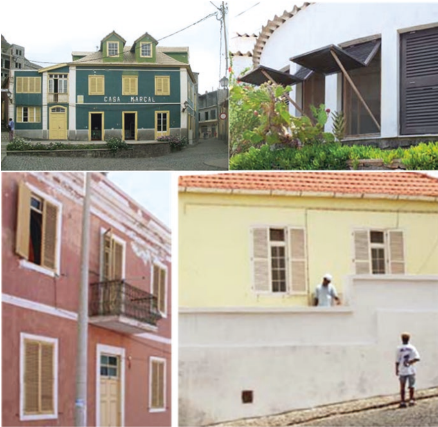
Fig. 3.65 External venetian blinds in Ribeira Grande and in Mindelo. As well as shading, they allow and direct the flow of natural ventilation
