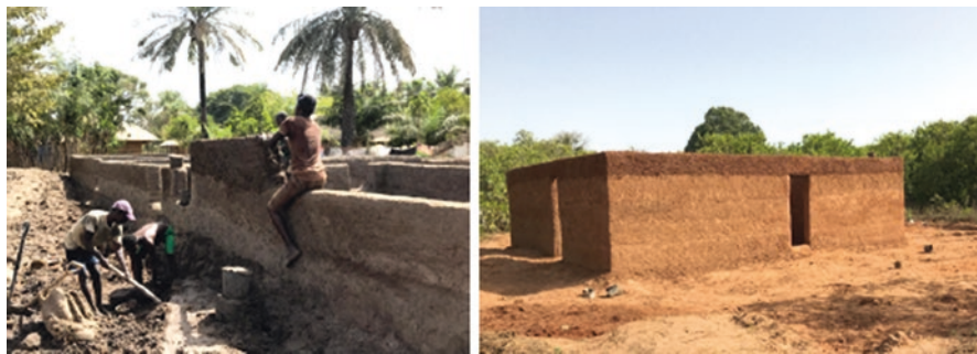
Figs. 3.120 and 3.121 Guinea – on the left, example of the construction process used in the Modelled Earth technique. On the right, example of dwelling built with this technique, clearly noticing the different construction levels still drying
