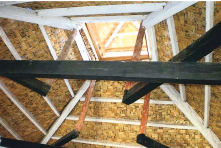
Fig. 3.88 Interior of a stack ventilation tower in a house in Sao Vicente
