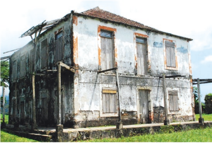
Fig. 13.5 Ordinary rubble masonry walls in a S. Tomé plantation building
