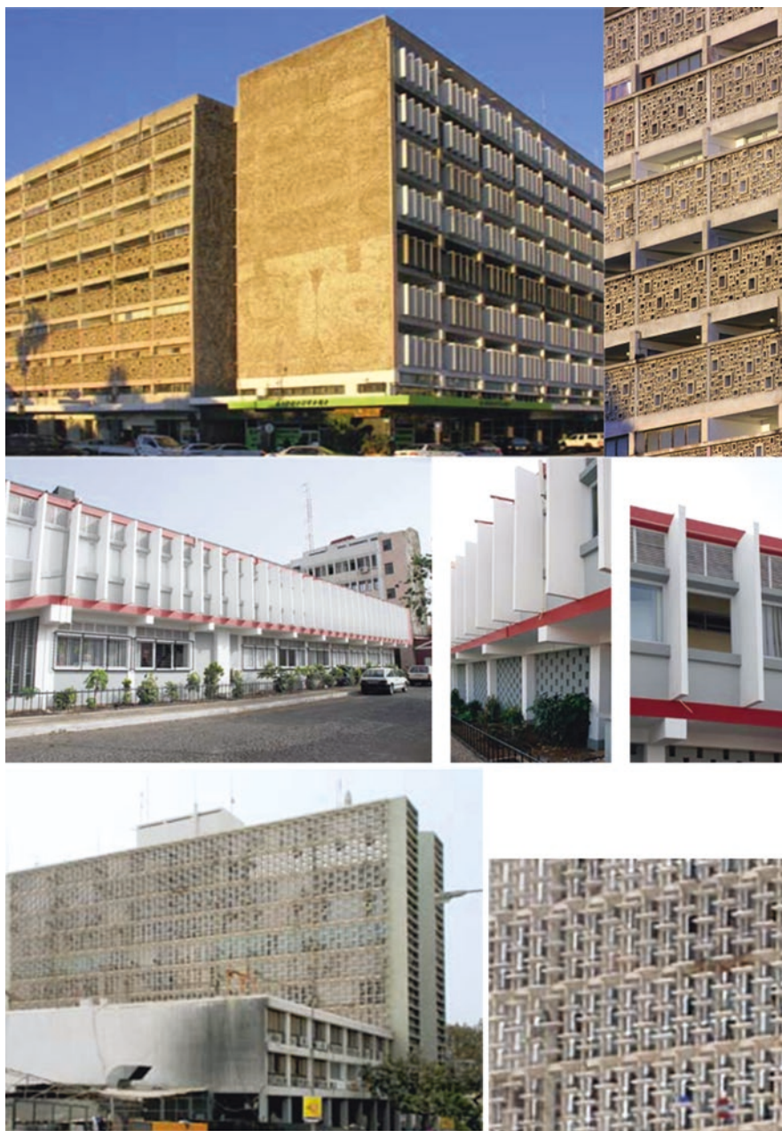
Fig. 3.27 Use of fixed shading devices (“Brise-soleil”) in modernist buildings in Maputo (Mozambique, above); in Praia, Cape Verde (centre); and in Luanda, Angola (below)
