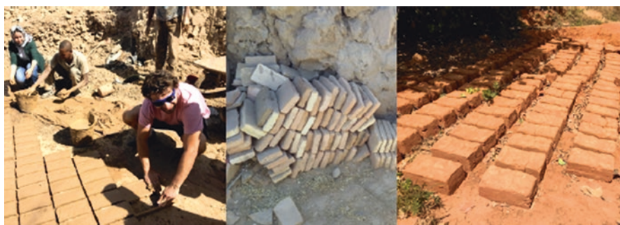
Figs. 3.125, 3.126 and 3.127 Morocco and Guinea – on the left, example of Moulded Adobe technique; on the centre, stack of blocks used for construction; on the right, Moulded Adobe blocks drying in the sun, showing that same technique can produce different blocks
