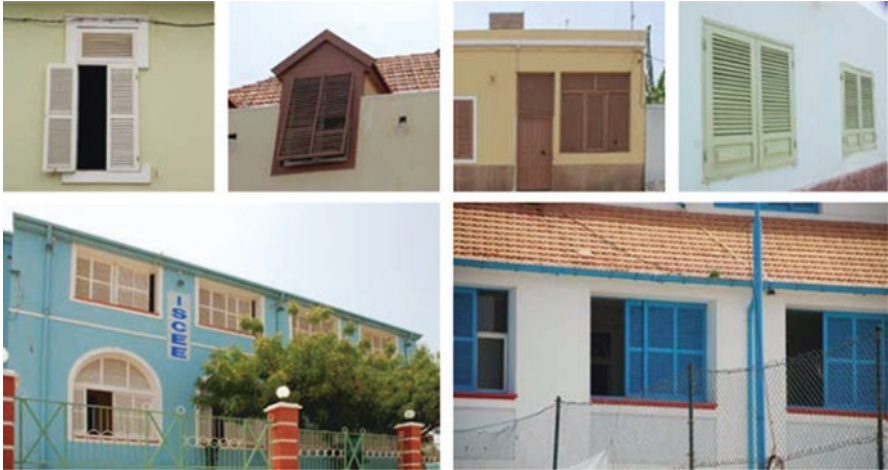
Fig. 3.71 External shutters are a typology traditionally used in Cape Verde and Bissau. They provide window shading and allow the control of the natural ventilation flow to the interior of the building
