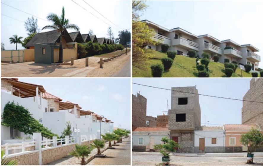
Fig. 3.18 On top (1) residential areas in Maputo, Mozambique: the twinning of houses reduces the area of sun exposure, reducing the risk of overheating. Below (2): left, geminated houses in Sal, Cape Verde; right, a dominant facade of an area contributes to situations of discomfort from overheating
