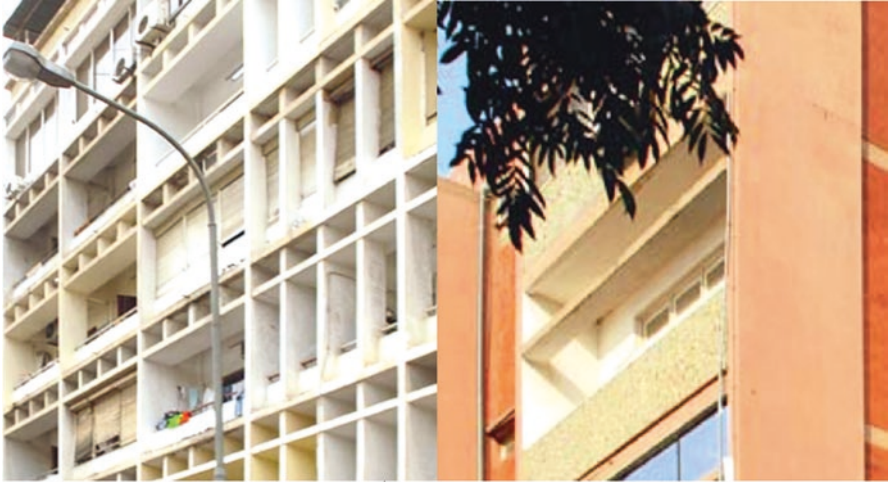
Fig. 3.30 Fixed shading in the facades of modernist buildings in Luanda
