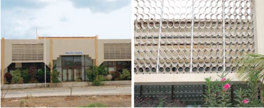
Fig. 3.33 Fixed shading in Cape Verde: double facade shading system, in an institutional building in the city of Praia. The exterior facade shades the glass and opaque areas through the use of an ingenious grid system using overlapping tubes, allowing for natural light and ventilation
