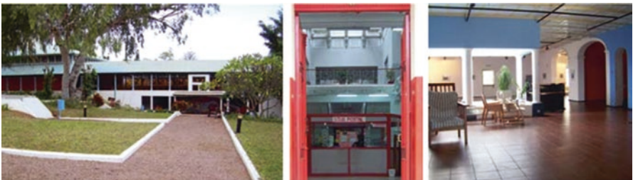
Fig. 3.79 Ventiladed atria in two buildings, Maputo, Mozambique
