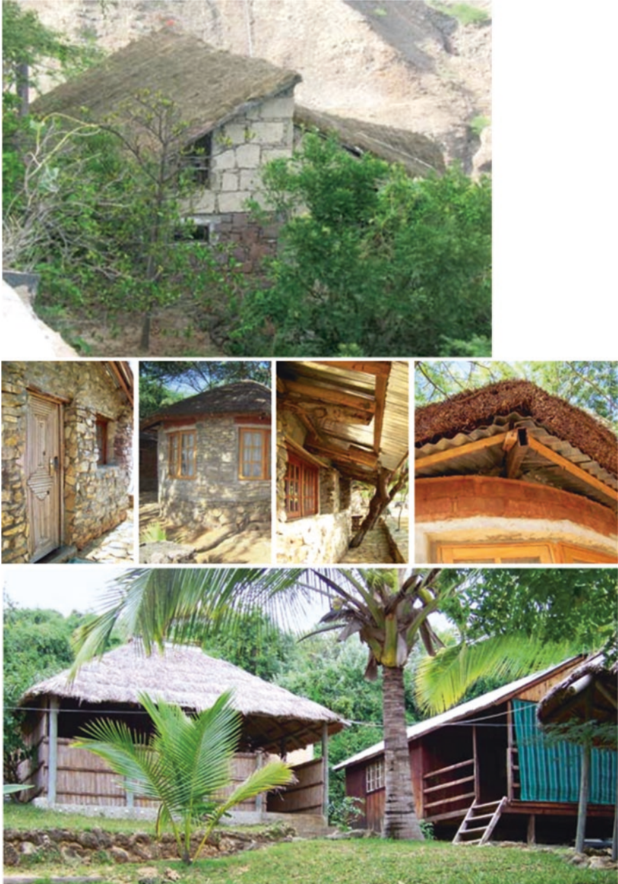
Fig. 3.6 Above: vernacular house in Santo Antão, Cape Verde, adapted to the climatic context. Below: buildings in a recent tourism complex, with building typologies inspired in vernacular architecture, in Angola (centre) and Mozambique (bottom)
