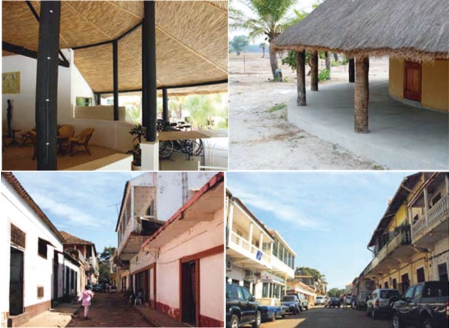
Fig. 3.38 Fixed shading: (above) shading projection of roof in a contemporary residential building in Guinea-Bissau. Below: shaded streets in Bissau
