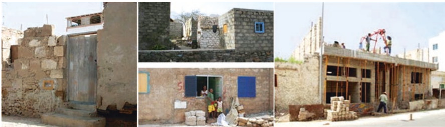
Fig. 3.106 New construction (above) and traditional, popular construction (below) in Cape Verde, using massive materials
