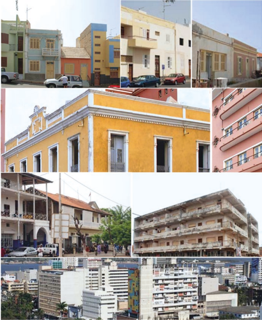
Fig. 3.62 Most residential buildings we find in more established urban areas in Cape Verde (above), Angola (centre), Guinea (below) and Mozambique (bottom) have very reasonable glazing areas. They are a good reference for the design of new buildings. The area of glass should not exceed 30% of the total area of the main facade and should be fully shaded
