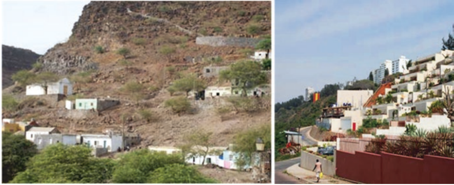
Fig. 3.7 Left: mountainside houses on the island of Santo Antão, Cape Verde. Right: recent residential condominium located in a slope, in Maputo, Mozambique
