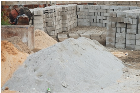
Fig. 13.7 Manufacturing of concrete blocks in S. Tomé Island
