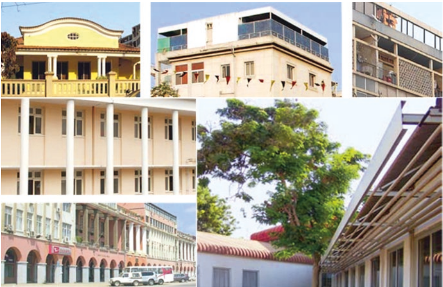
Fig. 3.31 Fixed shading in Luanda. Above: porch (left), shaded roof (centre), “Brise-soleil” (right). Below: arcades (left) and a fixed shading device at the Faculty of Architecture’s building (right)
