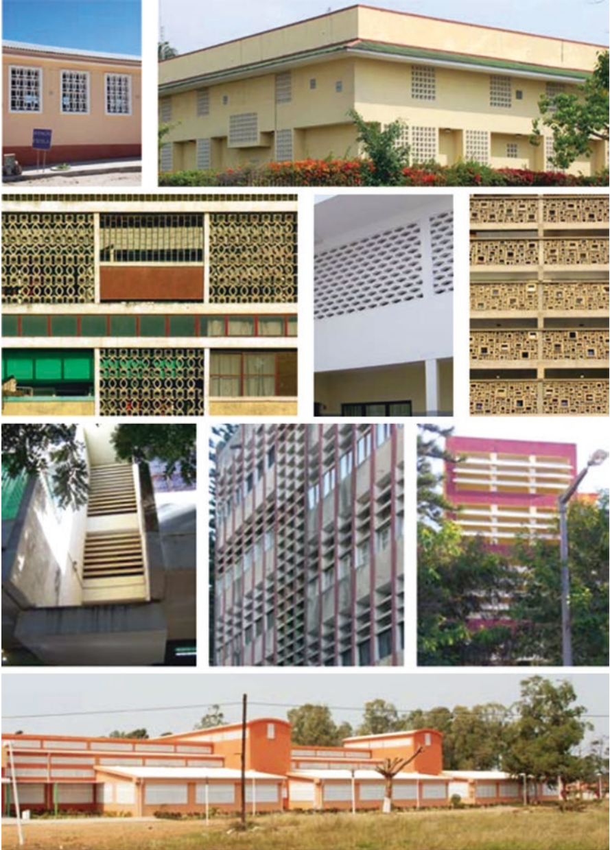
Fig. 3.69 “Brise-soleil” grills in Mozambique, for shading and natural ventilation
