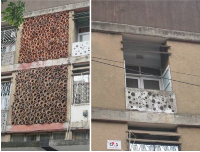
Fig. 6.29 The building for housing dockers
