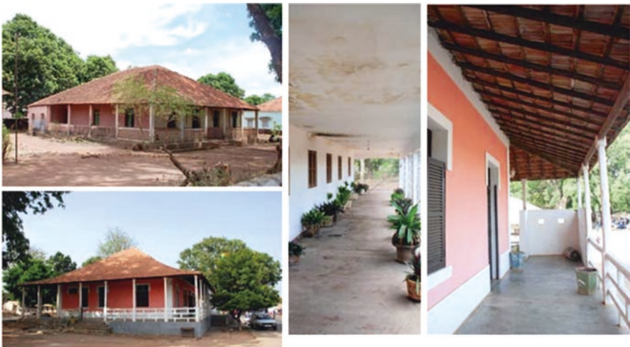
Fig. 3.37 Examples of shaded porches in colonial buildings in Guinea-Bissau
