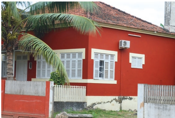
Fig. 13.11 Effects of rising dampness in a building in S. Tomé island
