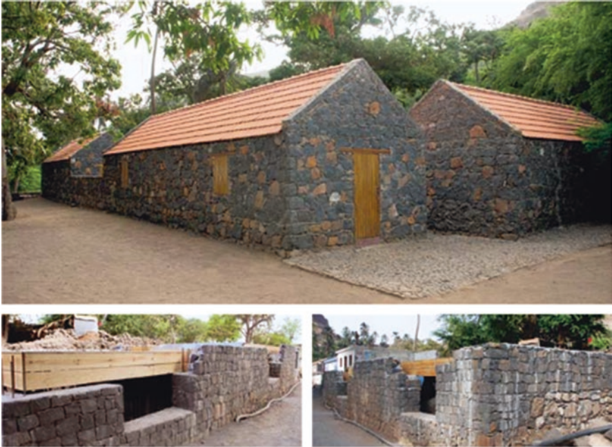
Fig. 3.107 Hostel designed by Alvaro Siza in Cidade Velha. New constructions using materials with high thermal inertia (stone and concrete)
