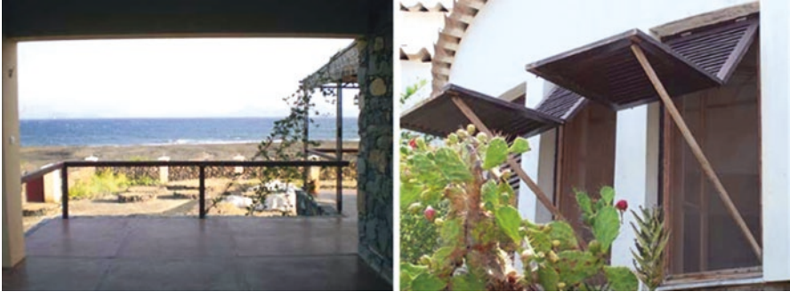
Fig. 3.23 Left: a house with covered courtyard in Porto Novo. Right: adjustable external shading in a house in Mindelo, Cape Verde
