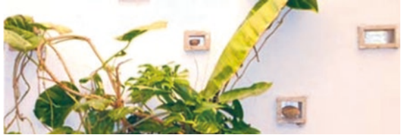
Fig. 3.76 Vents with mosquito nets in a house in Mindelo
