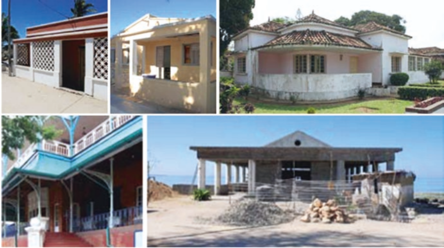
Fig. 3.42 Shaded porches, Mozambique
