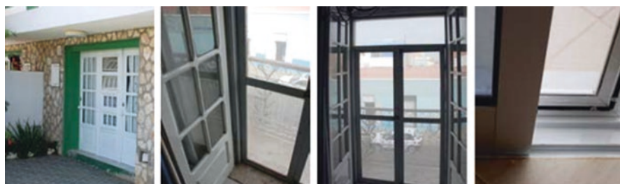
Fig. 3.75 Windows protected with mosquito net, in Praia
