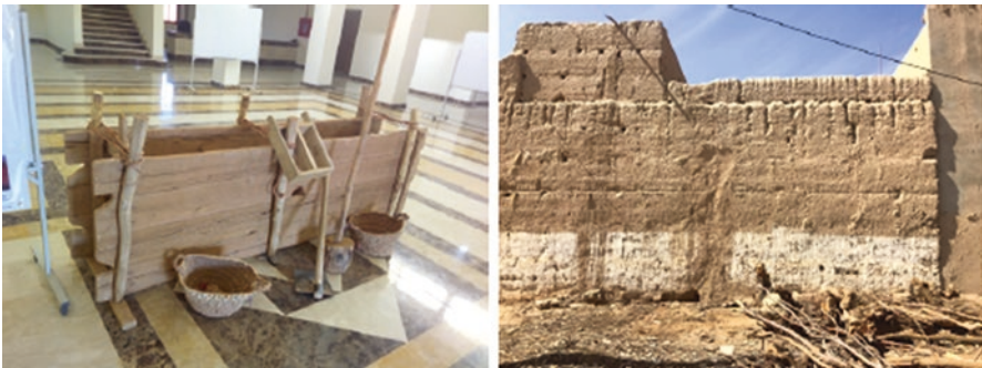
Figs. 3.118 and 3.119 Morocco – on the left, example of the formwood and other instruments used in the Pressed Earth technique. On the right, example of wall built with this technique, clearly noticing the holes resulting from the formwork and the different construction levels
