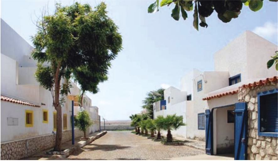
Fig. 3.20 Use of porches and vegetation canopies for protection against solar radiation in residential buildings (Cape Verde)
