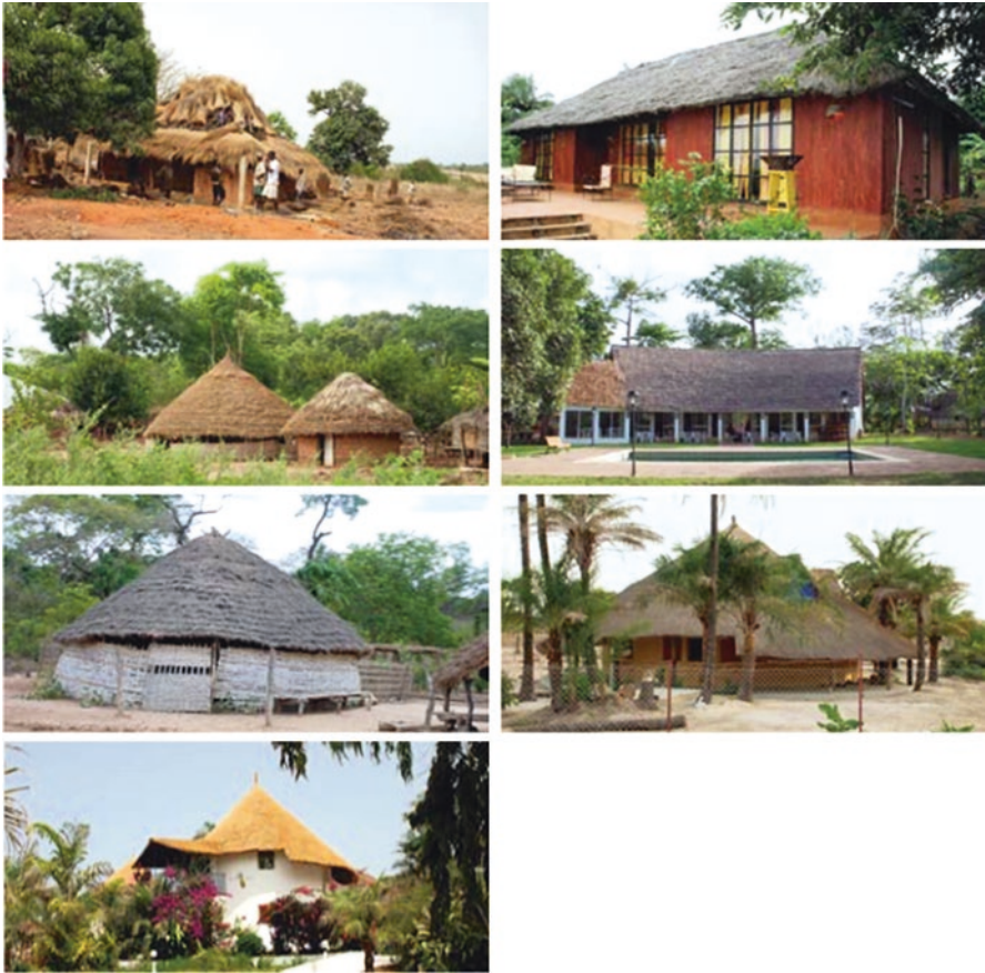
Fig. 3.58 Use of thatch in vernacular (left) and contemporary (right) buildings, in Guinea-Bissau
