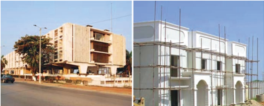
Fig. 3.50 Buildings painted white, in Luanda, Angola: the painting of buildings with light colours (e.g. using whitewash) would be an economical way to significantly reduce the discomfort from overheating
