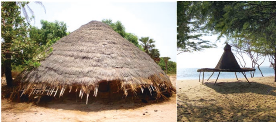
Fig. 3.22 Shading is a century-old heat protection technique. Vernacular buildings in Guinea-Bissau (left) and Angola (right)
