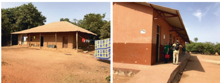
Figs. 3.134 and 3.135 Guinea – on the left, example of a more traditional house, more roughly built, but with attention to raising the floor; on the right, a more modern example of a more carefully built structure intended as a school, sharing the same solution
