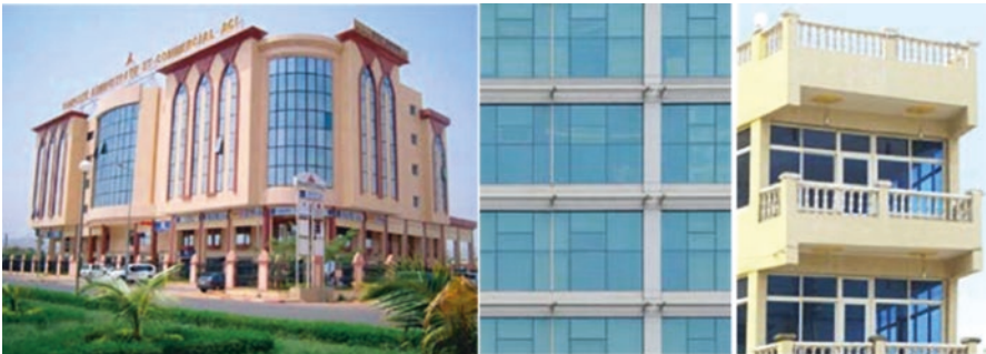
Fig. 3.5 Examples of imported architectural typologies, inadequate to the local climatic and social-economic context (Bissau, left; Luanda, centre, right)
