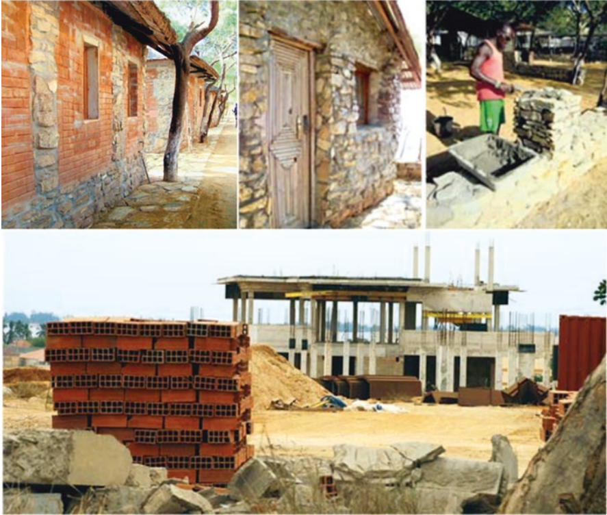
Fig. 3.105 New construction near Luanda, using massive materials – brick, stone and concrete – which provide thermal inertia to the building. This type of construction is adequate to hot climates with significant amplitudes between daytime and night-time temperatures
