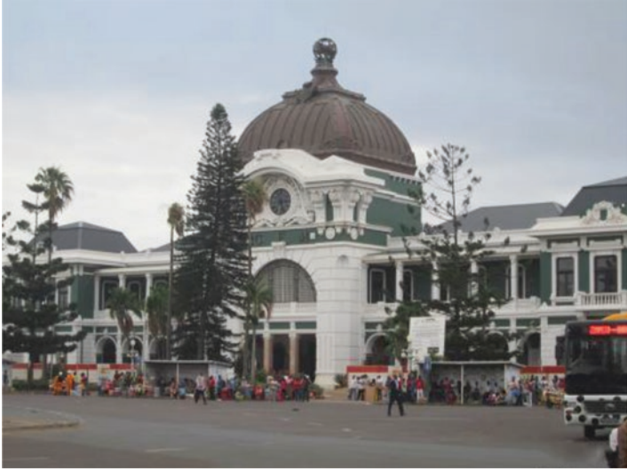
Fig. 6.4 Central railway station
