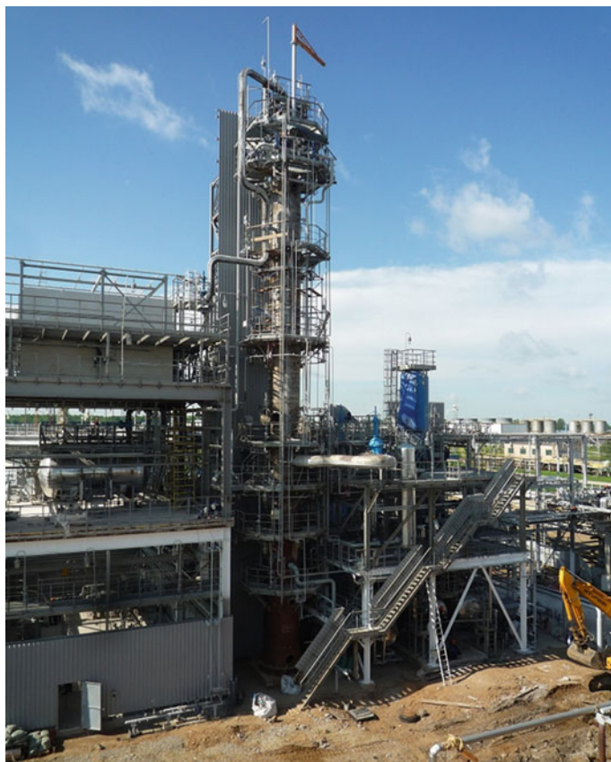
Fig. 1 General view of the new column during installation
