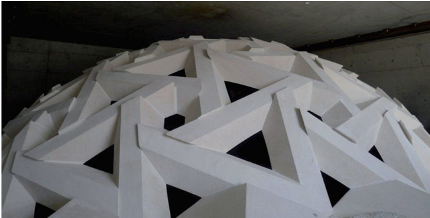
Fig. 14.14 Extrados of the Bin Jassim Dome, Doha, 2012
