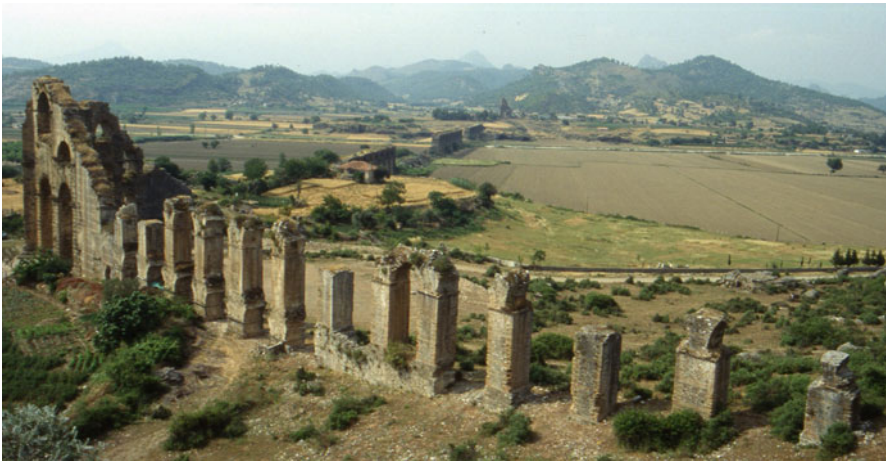
Fig. 2.17 The Stone-pipe inverted Siphon of Aspendos, on Arched bridge as Venter. (Photo by U. Ozis)
