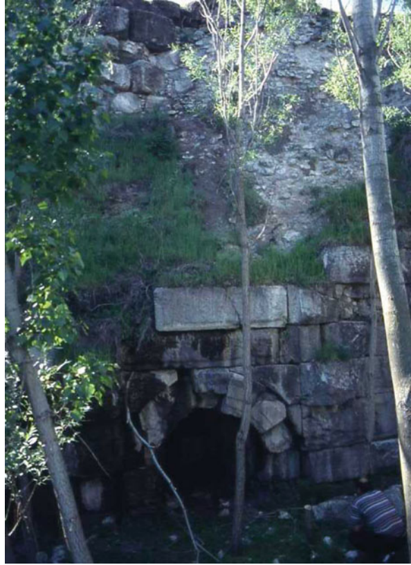
Fig. 2.24 The bottom outlet of the Orukaya Dam. (Photo by U.Ozis)
