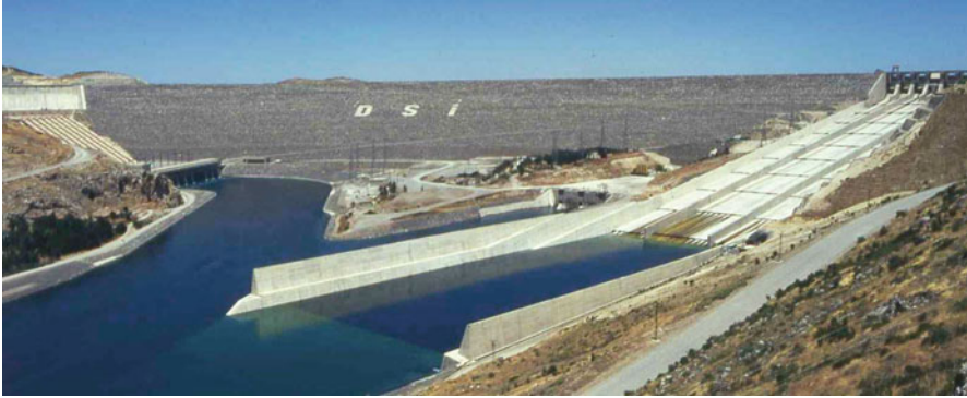
Fig. 12.19 The Ataturk dam on Euphrates. (Photo by U. Ozis)
