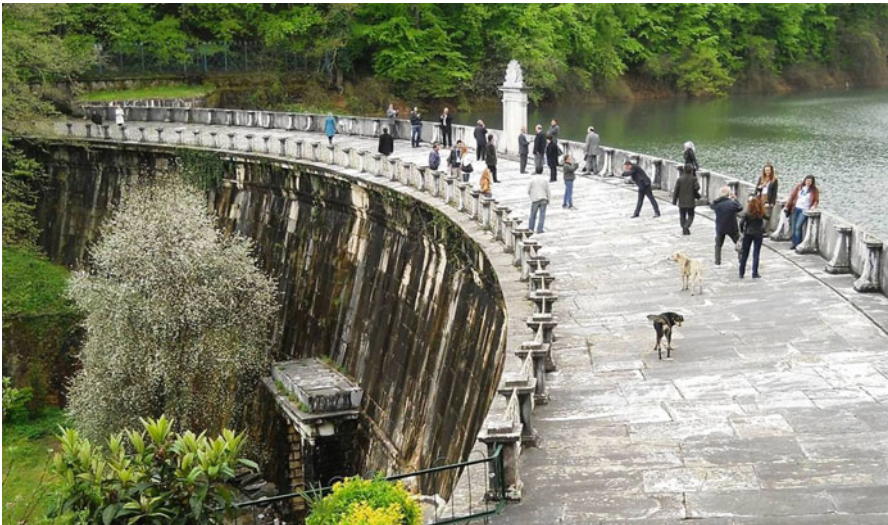
Fig. 2.31 Yeni Dam supplying the Taksim system. (Photo by Y.Ozdemir)
