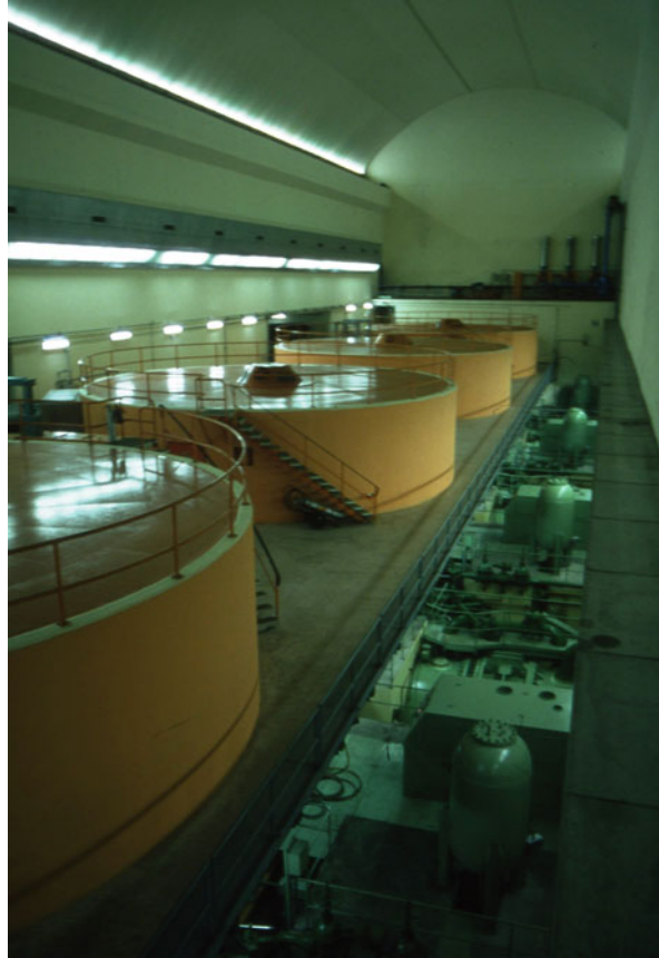
Fig. 10.17 Oymapinar underground powerhouse. (Photo by U. Ozis)
