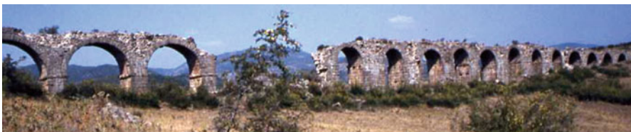
Fig. 2.5 The Roman Aqueduct-bridge of the Madradag Water Conveyance crossing the last valley before Pergamon. (Photo by U.Ozis)
