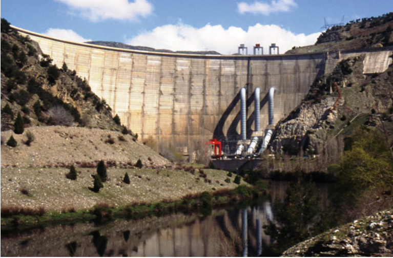
Fig. 10.9 Gokcekaya dam and power plant of 300 MW on Sakarya (intakes on the dam body). (Photo by U. Ozis)
