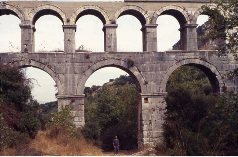
Fig. 2.8 The Sextilius Pollio Aqueduct-bridge on the Derbentdere Water Conveyance to Ephesus. (Photo by U.Ozis)
