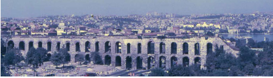
Fig. 2.4 Valens (Bozdogan) Aqueduct-bridge in Constantinople (Istanbul). (Photo by U.Ozis)
