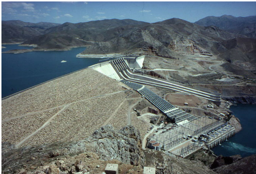
Fig. 10.18 Keban embankment dam on Euphrates and the 1330 MW power plant. (Photo by U. Ozis)
