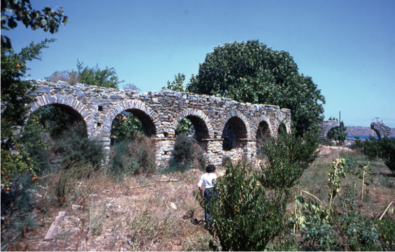
Fig. 2.14 The Aqueduct-bridge in Iasos. (Phot by U.Ozis)
