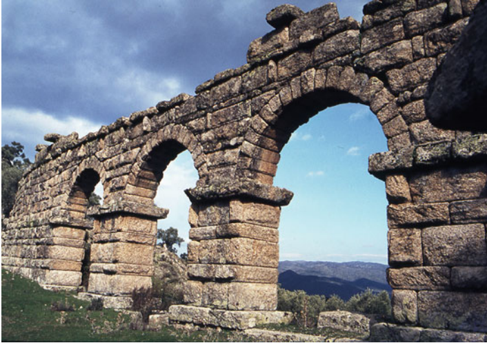
Fig. 2.12 The last Aqueduct-bridge of the water conveyance to Alinda. (Photo by U.Ozis)
