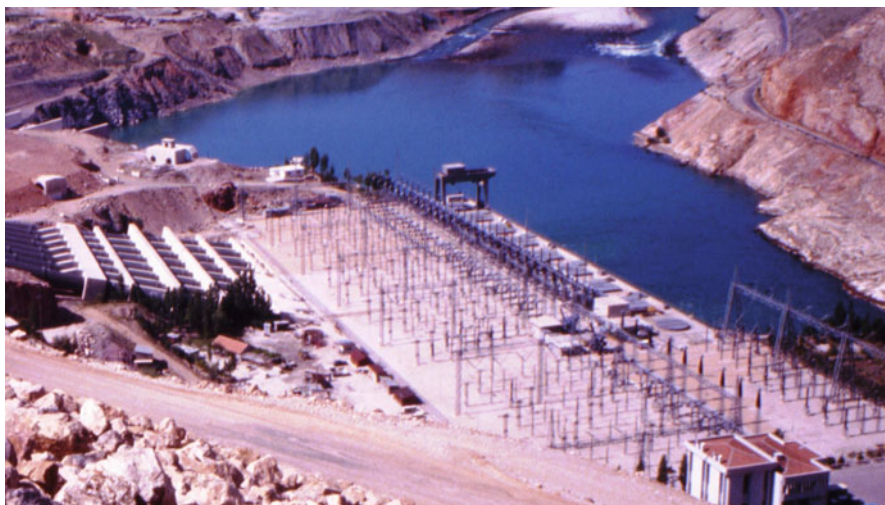
Fig. 10.16 Keban semi-outdoor type powerhouse. (Photo by U. Ozis)
