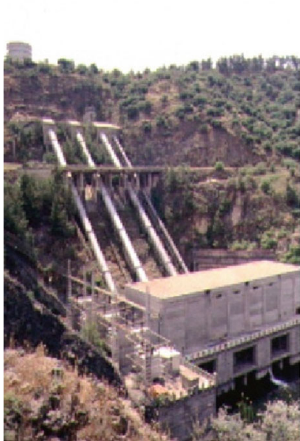
Fig. 10.5 Demirkopru diversion scheme, with 107 m head (fed from the embankment dam on Gediz river by the 2.4 km long pressure tunnel), surge tank, penstocks, and powerhouse. (Photo by U. Ozis)
