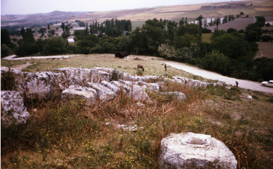
Fig. 2.10 Stone-pipe inverted Siphon of the water conveyance to Laodicea. (Photo by U.Ozis)
