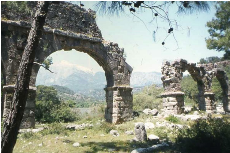
Fig. 2.16 The Aqueduct-bridge in Phaselis. (Photo by U.Ozis)
