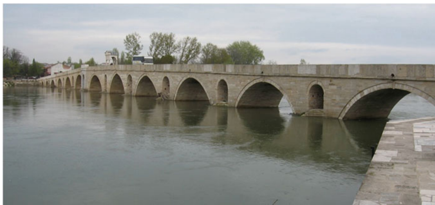
Fig. 12.4 Maritza (Meric) River and the 263 m long Mecidiye Bridge (1847) in Edirne. (Photo by U. Ozis)
