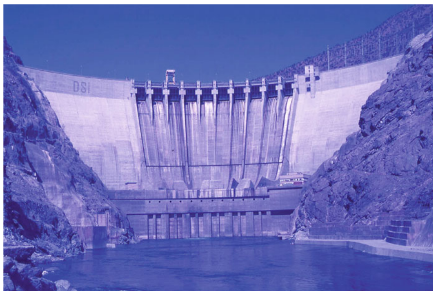
Fig. 10.4 Karakaya arched gravity dam and power plant of 1800 MW capacity on Euphrates. (Photo by U. Ozis)
