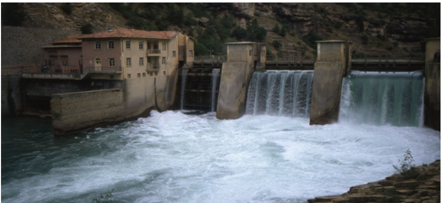
Fig. 10.7 Low-head, run-of-river Maras hydroelectric plant, of 3.6 MW, on Ceyhan river. (Photo by U. Ozis)
