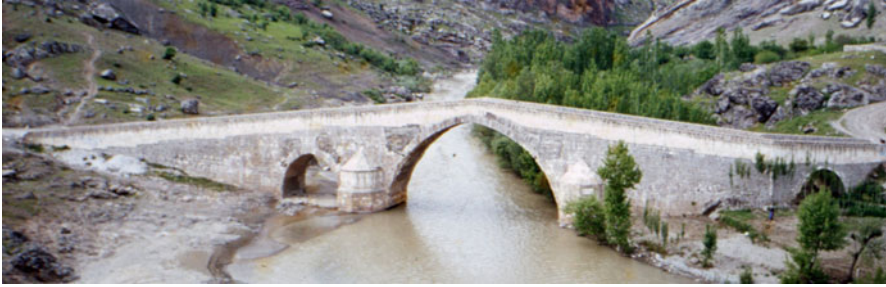
Fig. 2.25 A Canal, supplying a water Mill, through the Seljukide Haburman Bridge in Cermik. (Photo by U.Ozis)
