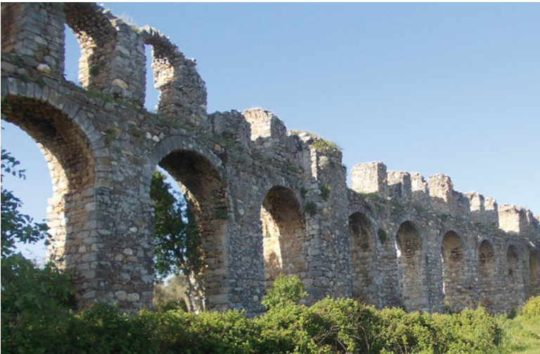
Fig. 2.15 The 2.3 km long Aqueduct-bridge in Mylasa. (Photo by A.Alkan)
