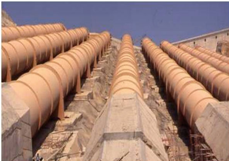
Fig. 10.12 Penstocks of the Ataturk power plant with diameters of 7.5–6.6 m. (Photo by U. Ozis)
