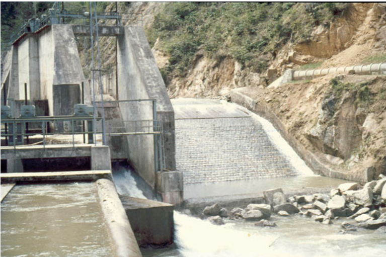
Fig. 10.10 Ikizdere high-head diversion scheme on Iyidere, diversion weir and frontal intake (Photo by U. Ozis)
