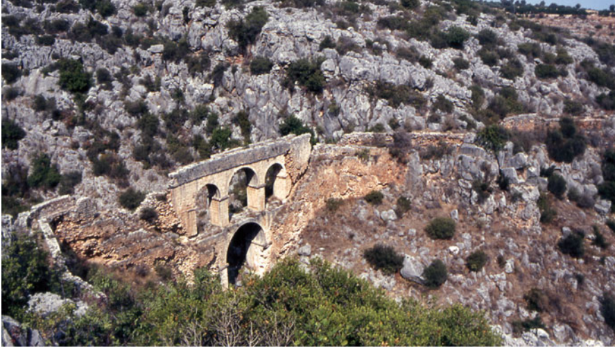
Fig. 2.19 Kumkuyu Aqueduct-bridge of the water conveyance to Elaiussa Sebaste. (Photo by U. Ozis)
