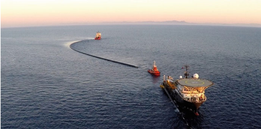
Fig. 3.9 Installation of pipes. (DSI 2018c)
