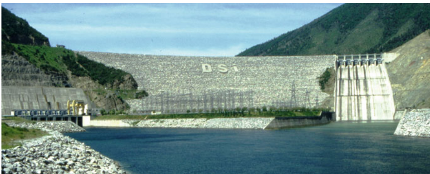
Fig. 10.8 Altinkaya dam and power plant of 700 MW on Kizilirmak (intakes at the right abutment). (Photo by U. Ozis)
