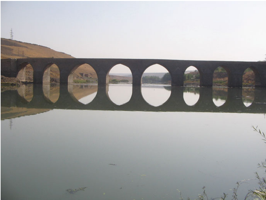
Fig. 12.16 The Tigris River near Diyarbakir with the 180 m long Dicle-Bridge of roman origin. (Photo by A. Alkan)
