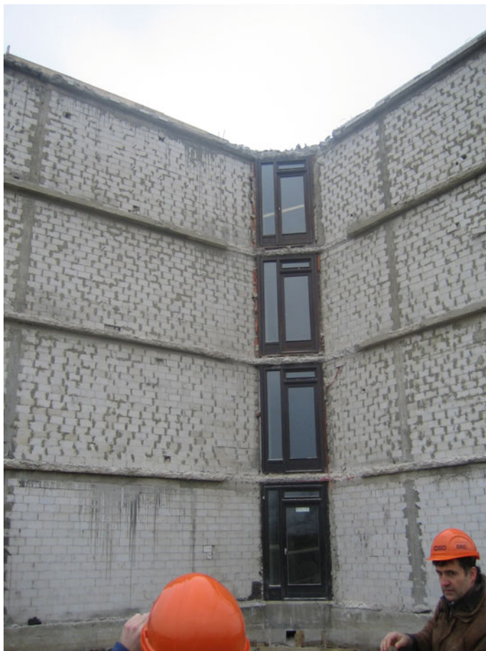
Fig. 4.23 Hotel Terme Čatež prior to structural upgrade [108]
