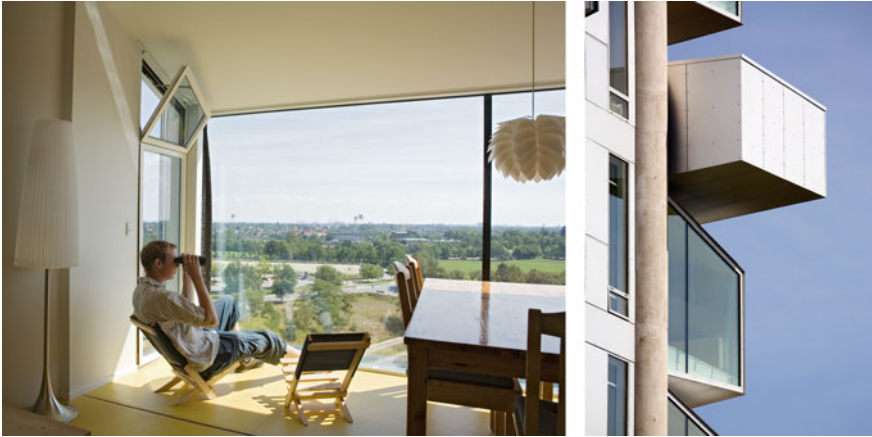
Fig. 2.12 Along with unimpeded views the added crystal-like bay windows enlarge the usable floor area and emphasize the refreshed aesthetics as also the added function of the renovated building (photographs by Torben Eskerod)
