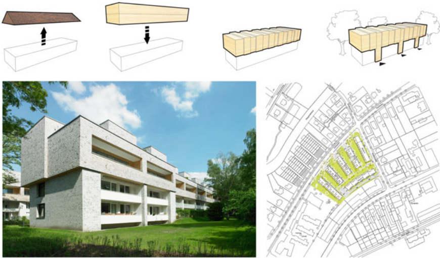
Fig. 2.9 Urban densification of a residential district located at the edge of the Hamburg city by means of vertical building extension (photograph by Martin Lukas Kim, drawings by blauraum)
