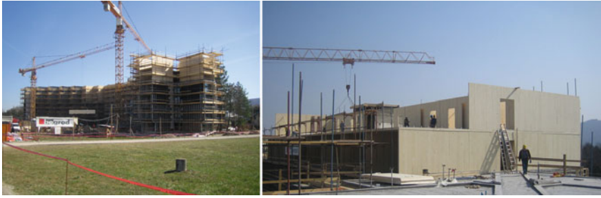
Fig. 4.24 Hotel Terme Čatež during the construction of the two-storey CLT upgrade module [108]
