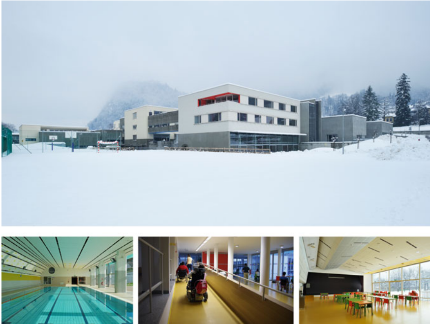
Fig. 2.7 Renovated Centre for education and rehabilitation of physically handicapped children and adolescents CIRIUS in Kamnik, Slovenia (photos by Miran Kambič)
