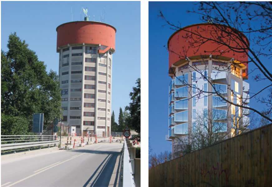
Fig. 2.11 Jægersborg Water Tower prior to (left) and after (right) the conversion (photograph by Dorte Mandrup and Jens Markus Lindhe respectively)
