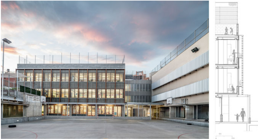
Fig. 2.5 A new south façade enables multiple functions next to the energy performance improvement (photo by Adrià Goula, drawing by HARQUITECTES)
