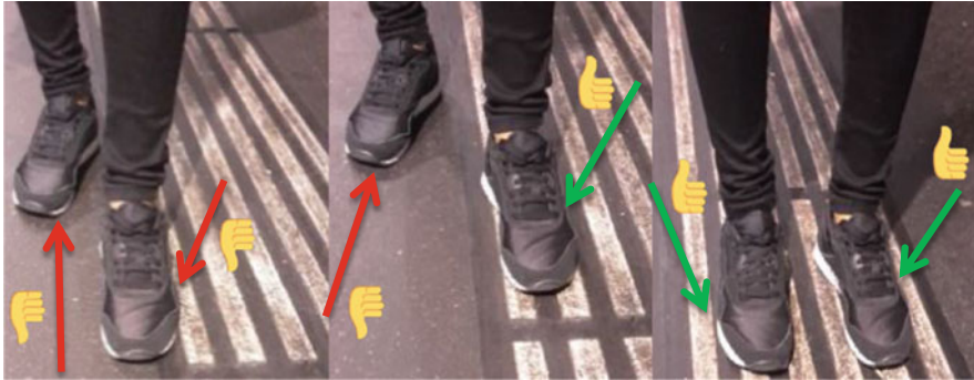
Fig. 2 Safety line at platform of Bern (CH); red arrow is “in danger zone”—indicator
