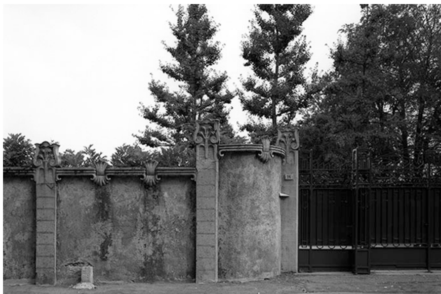
Fig. 2 Wall fence of Villa Mauri. Gallarate (VA)
