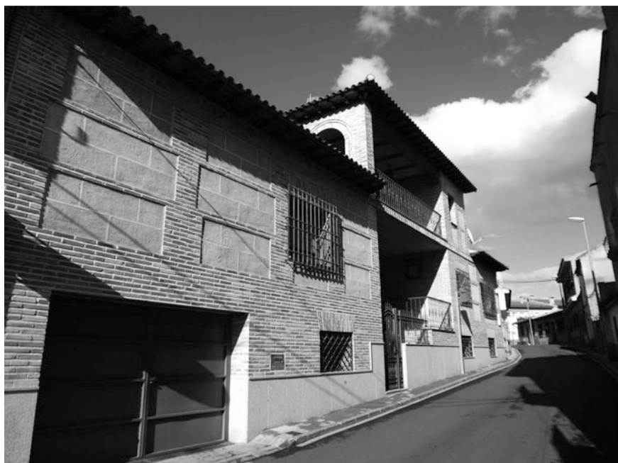
Fig. 16 Recently built houses in Bargas, showing unsuccessful attempts to imitate local aparejo toledano walls
