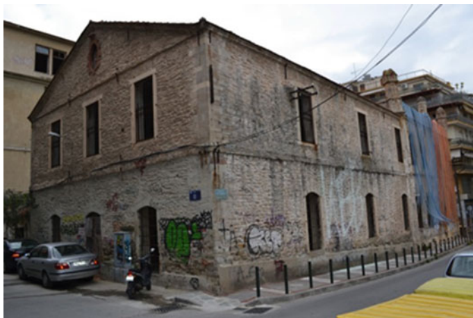
Fig. 8 The first offices of M.L. Herzog et Cie, built after 1891 (© Ivkowska, 2015)
