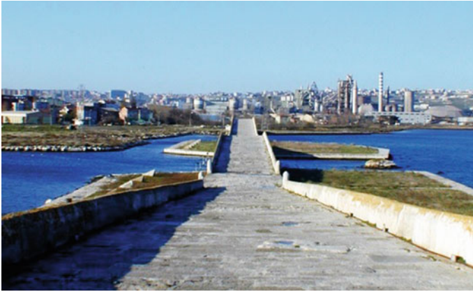
Fig. 13 The bridge and its environment today (© Orlandi)
