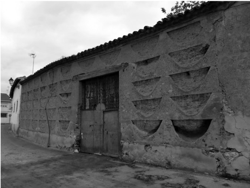
Fig. 9 Brenchas rammed earth wall in Carranque
