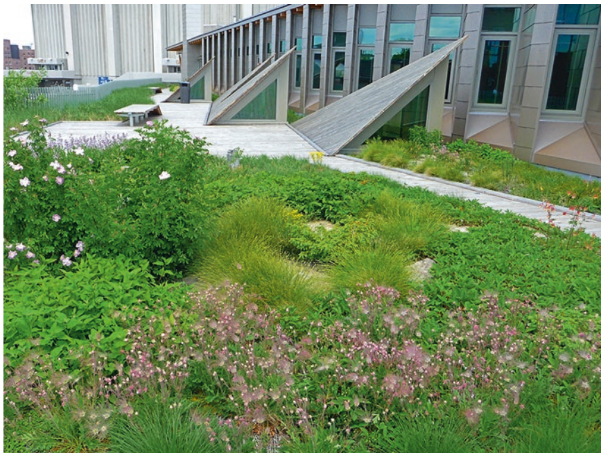
Fig. 15.10 The green roof at Gateway Center in Syracuse, NY. The image highlights the use of plants from native plant communities (alvar grassland and Eastern Ontario dune) that provide enhanced pollinator services throughout the year. (Source: Tim Toland)
