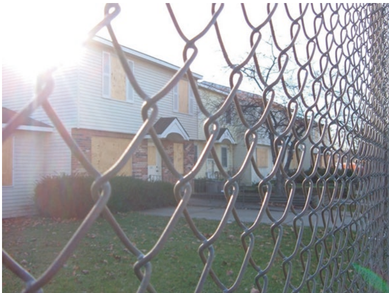
Fig. 13.1 Homes bordering Midland neighborhood park boarded up in preparation for construction of a regional sewage treatment facility. (photo courtesy of M. Hall)
