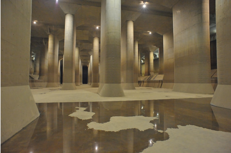
Fig. 16.1 A portion of the Metropolitan Area Outer Underground Discharge Channel in Tokyo © Flickr user “ptrktn” available from https://www.flickr.com/photos/ptrktn/3353015541
