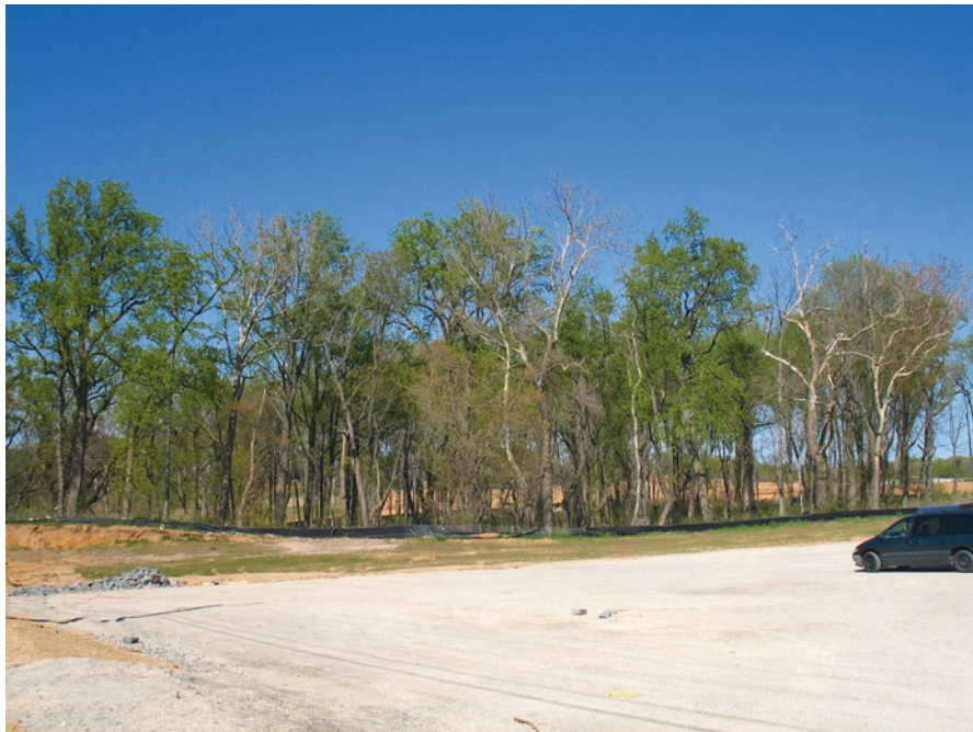
Fig. 15.2 Tree preservation areas are typically a component of site development and in some cases contribute to open space and stipulated tree coverage requirements. However, they are usually just fragments of a once larger ecosystem and that, combined with the stresses of construction activity, can severely compromise plant health and sustainability. (Source: Tim Toland)
