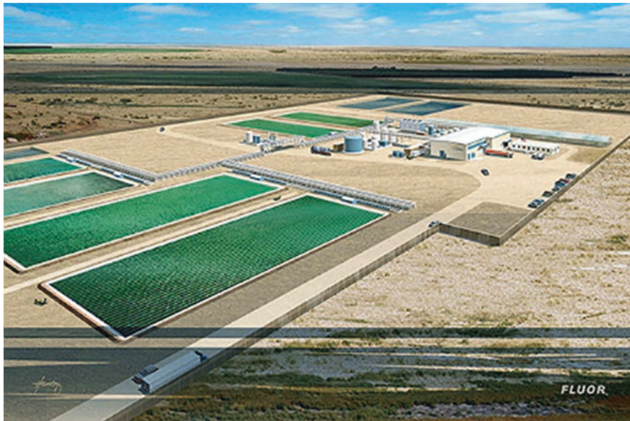
Fig. 12.29 Required system for the Kızıldere-I GPP (demonstration in Hobbs-New Mexico; https://www.chemicals-technology.com/projects/joule-sunsprings-biofuel-plant-new-mexico )
