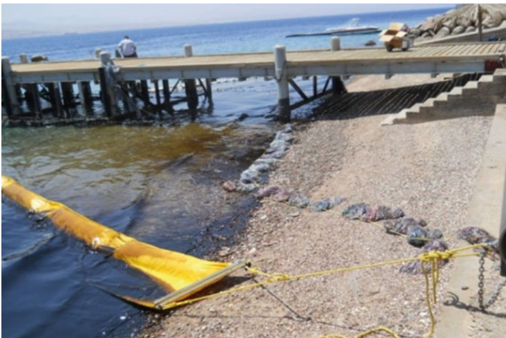
Fig. 15 Eilat Marine Pollution Station serving as “last frontier” to block and contain HFO pollution from MV AVRAMIT, 2012. Source: Eilat Marine Pollution Prevention Station, MEPD, Israel
