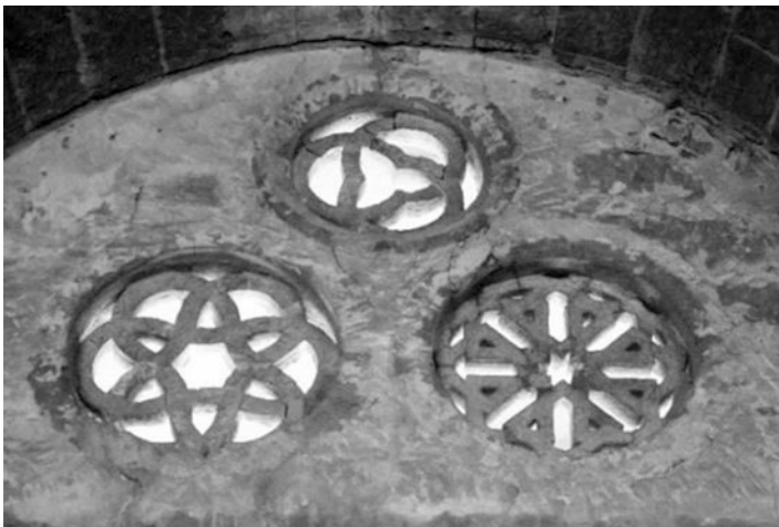
Fig. 8.4 Window with rosettes, south-east wall
