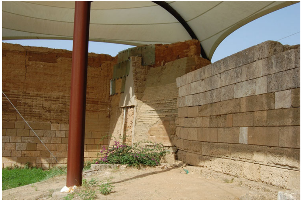
Fig. 5 Gela (archaeological site on the south coast of Sicily). Evidence of the subsequent conservational interventions on the earthen urban walls of Capo Soprano. Photograph by M.L.G. 2015
