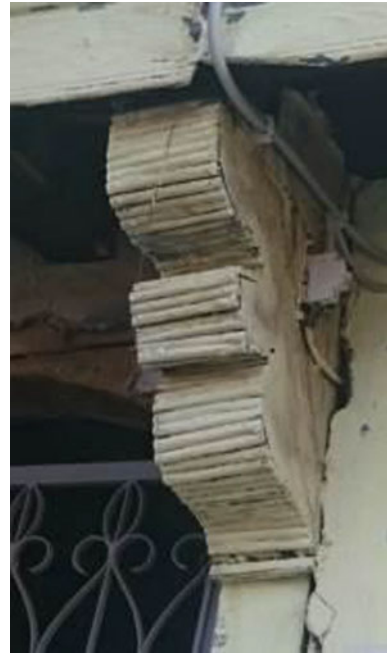
Fig. 45 A wooden buttress
