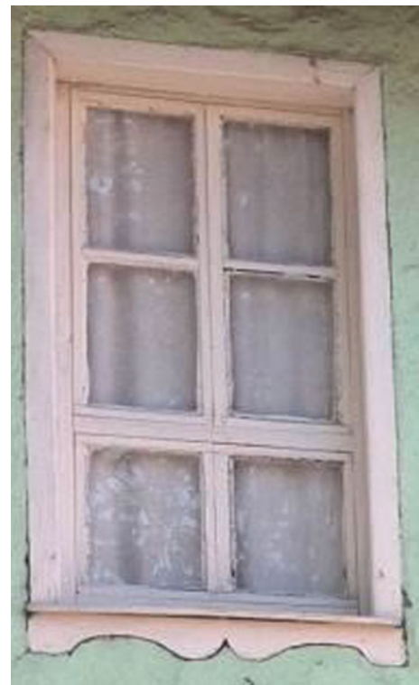
Fig. 41 Wooden window with two big and two small leaves
