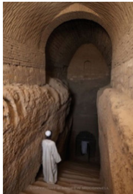
Fig. 7 Nubian vaults as the main design
