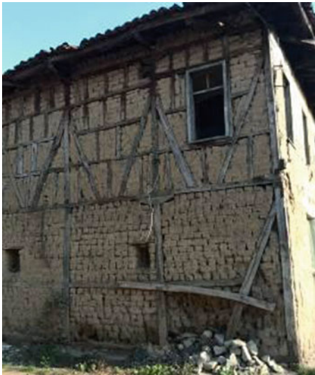
Fig. 26 Mudbrick wall and timber construction
