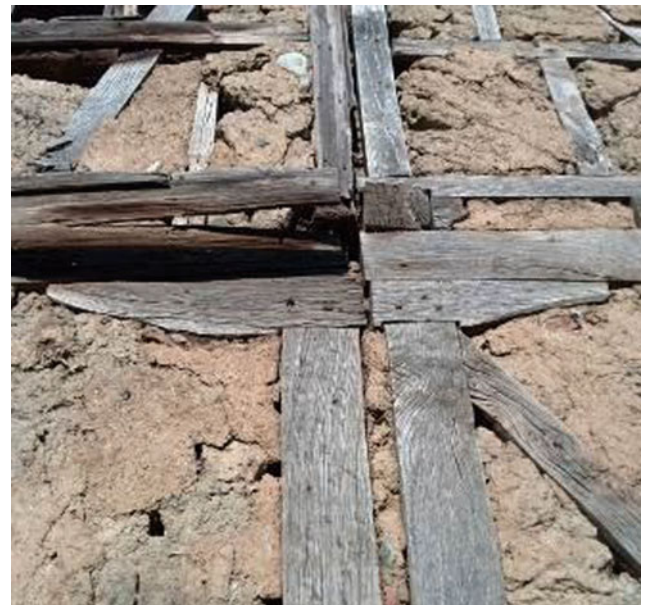
Fig. 29 Dilatation joint between two timber construction
