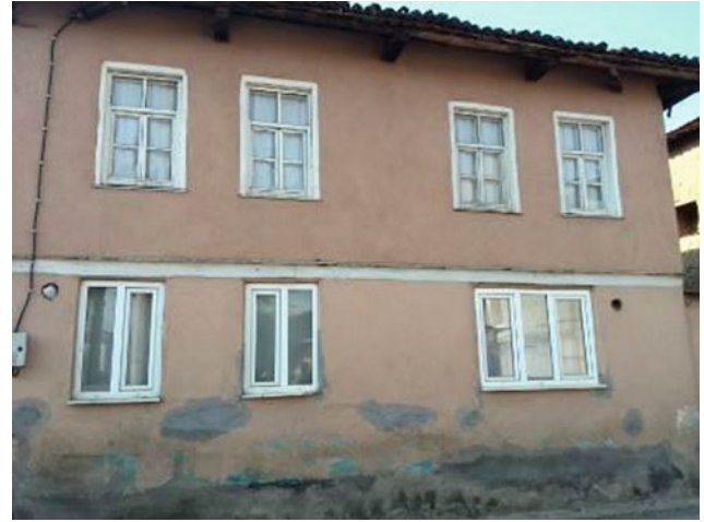
Fig. 48 New plastic windows and cement plaster on the wall
