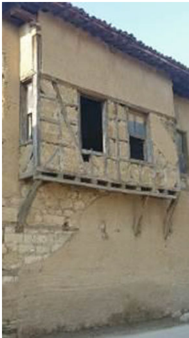
Fig. 43 Rectangular cantilever and wooden buttress
