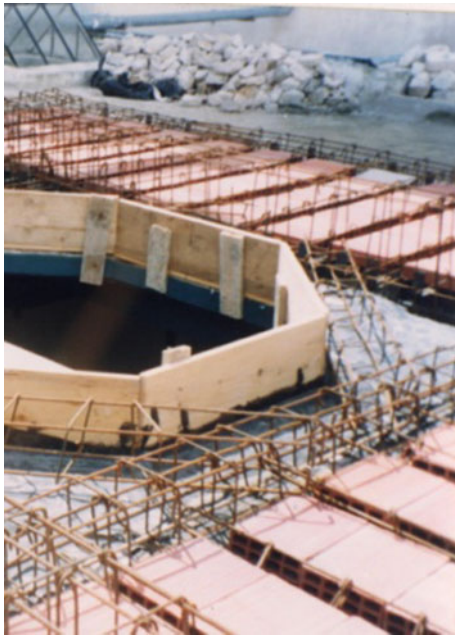
Fig. 24 Rebuilt slab of Dar Daouletli (Mouhli et al. 2013)
