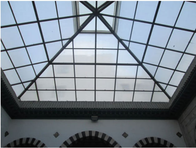
Fig. 28 Removable metallic roofing in Dar Daouletli (author's photograph)
