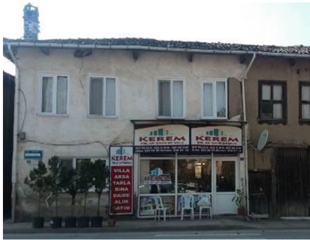
Fig. 47 New plastic windows on the first floor and the small shop arranged on the ground floor caused lost of authenticity
