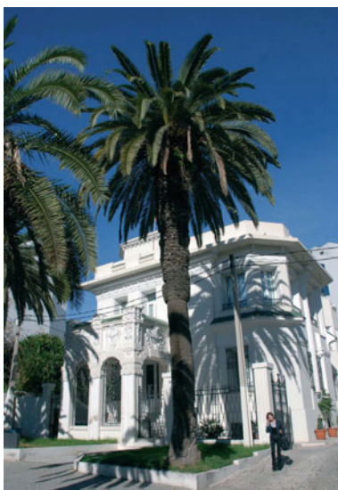
Fig. 7 Building before intervention (Khaled Ayed)
