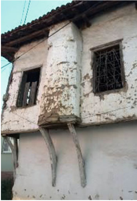
Fig. 46 Semicircular planned chimney arranged like a cantilever on the facade
