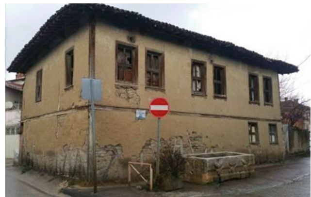
Fig. 12 Front facade of Building 7
