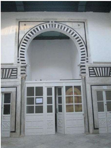
Fig. 29 Removable wood partitions in Dar Daouletli (author's photograph)
