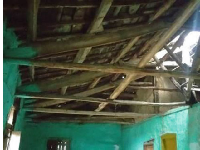
Fig. 32 Timber roof seen above the anteroom
