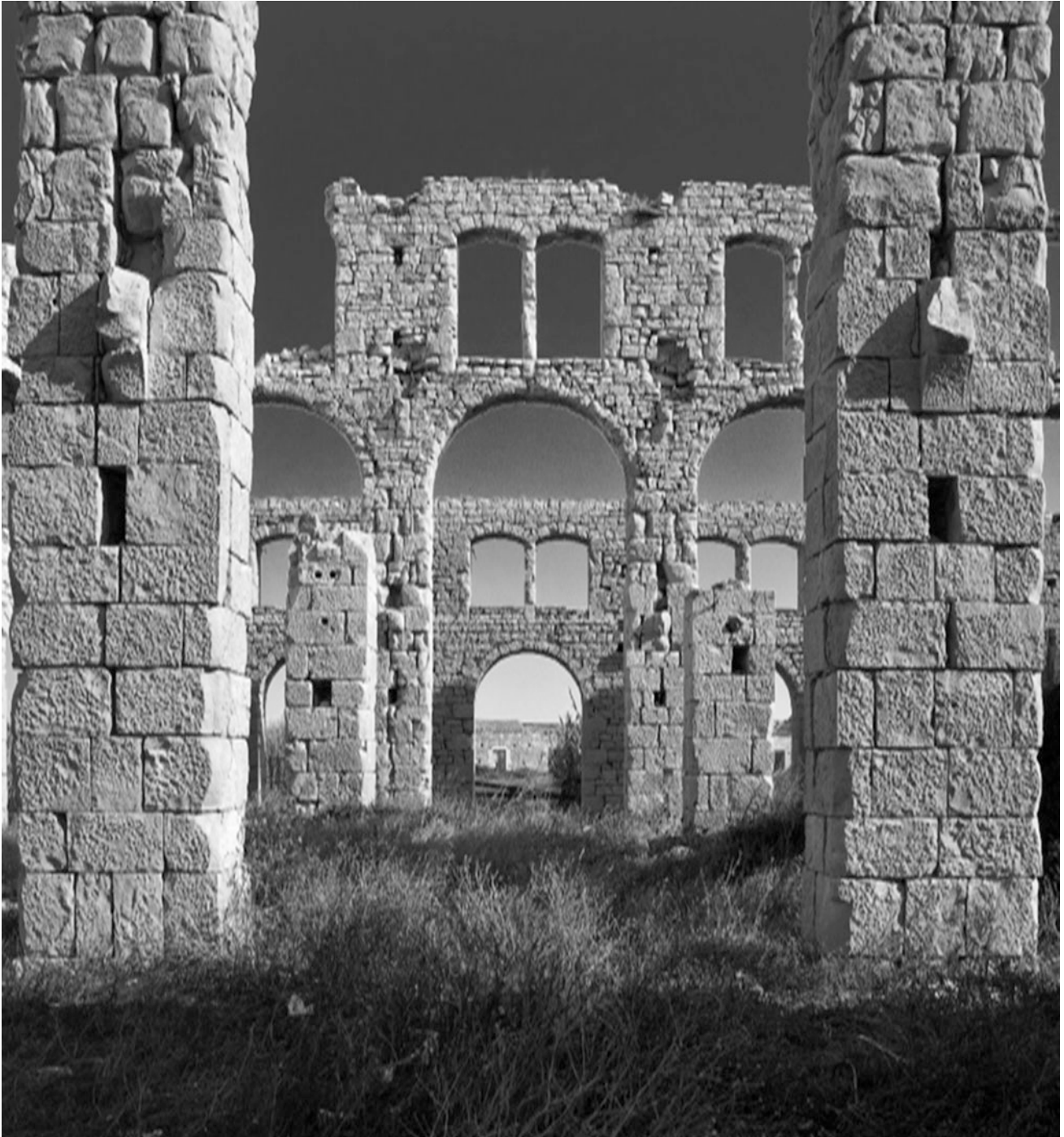
Fig. 3 Scicli, Penna brick factory. A detail of the dry masonry. Ph. Pasquale Bellia ( www.ragusaneews.com )
