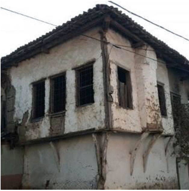
Fig. 42 Rectangular cantilevers arranged on both two facades supported with wooden buttress
