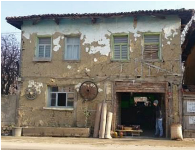
Fig. 19 Front facade of Building 7
