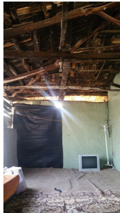
Fig. 25 Anteroom room at first floor
