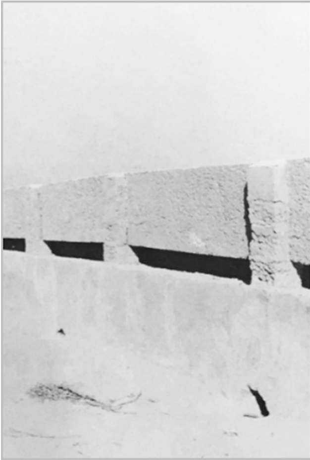
Fig. 17 Wind parapet (Lewcock 1978)
