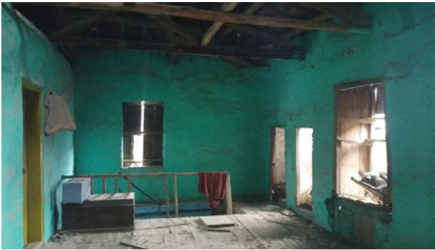
Fig. 14 Anteroom at the first floor
