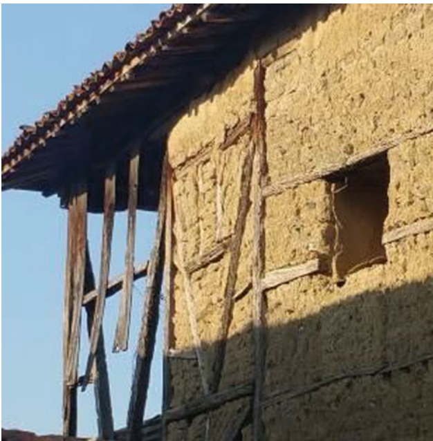
Fig. 27 Timber construction with mudbrick fillings
