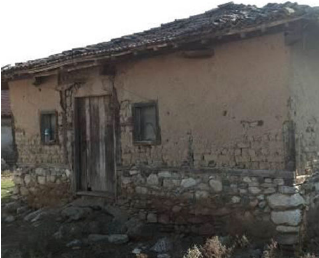
Fig. 35 Mudbrick walls of a stable
