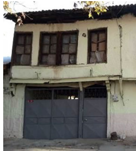
Fig. 49 New metal entrance door of the building
