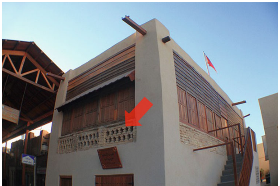
Fig. 28 Wall openings at Koshk Mubarak (Basel 2012)
