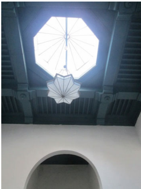
Fig. 25 Simple false ceiling in Dar Daouletli (author's photograph)
