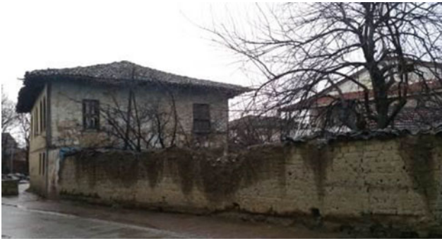
Fig. 13 Adobe garden walls of Building 7
