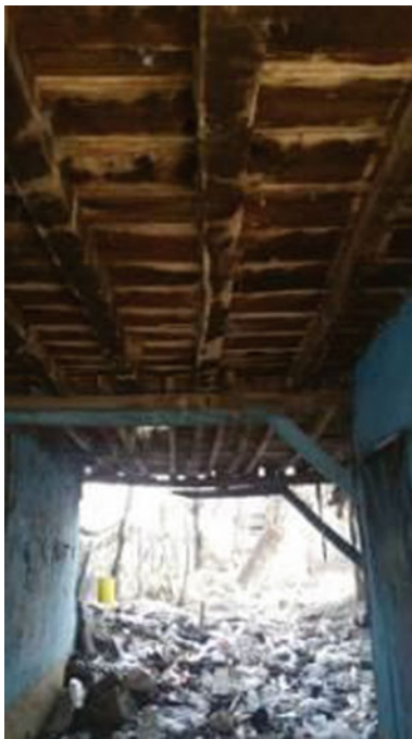
Fig. 31 Wooden beams on the ceiling
