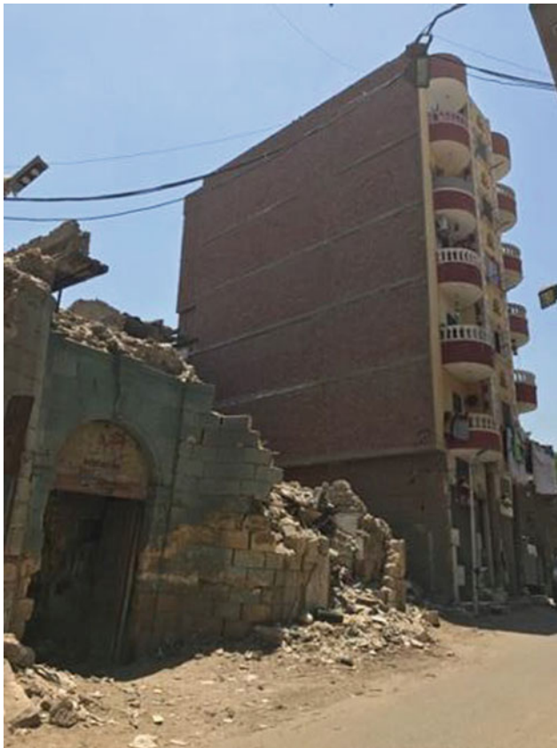
Fig. 2 A new informal building besides the distinguished building of “Beit Madkour” that was saved from demolishing by “Save Cairo”. Source Photograph by the Author in 2017
