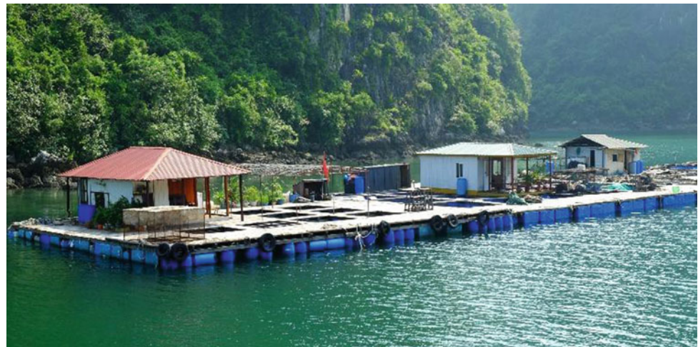
Fig. 8 A cluster of floating houses, Cat Ba island, Vietnam. Source Photographs taken by author 9-2016
