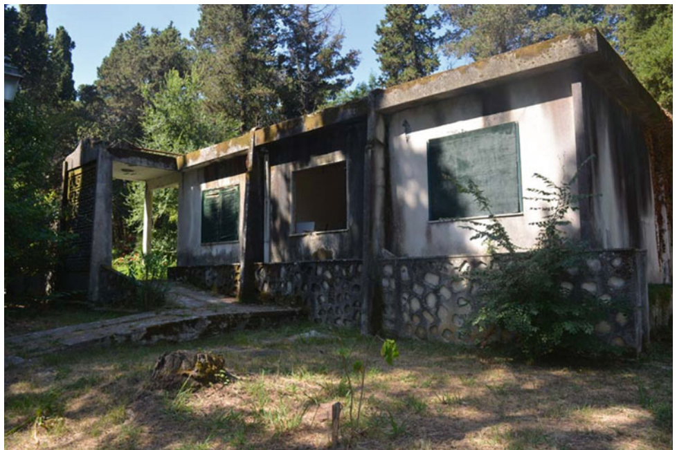
Fig. 5 Former clinic building, photo: Alexandra-Aikaterini Andrianou, April 2017
