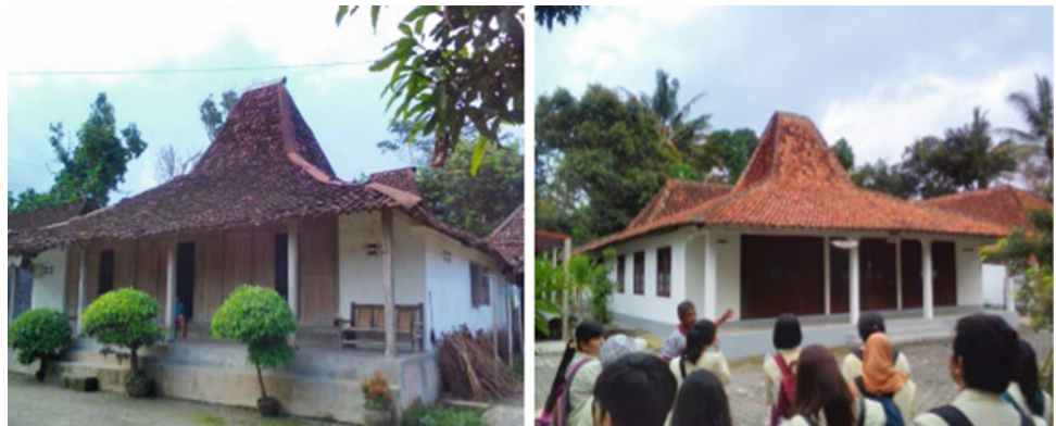
Fig. 1 Traditional Joglo House . Source Document survey, 2017
