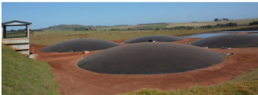
Fig. 5.7 Anaerobic co-digestion of swine carcass and manure. Source Monalisa Pereira
