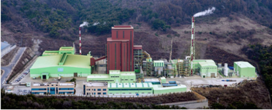
Fig. 5 View of GRM Plant [10]
