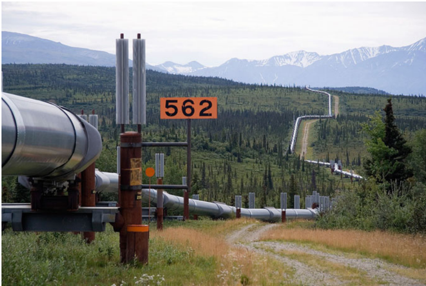
Fig. 4 Trans-Alaska pipeline with heat exchanger to protect permafrost from melting during the summer months (from: www.en.wikipedia.org/wiki/Trans-Alaska_Pipeline_System )
