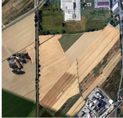
(a) Aerial view of the incinerator (source Google Earth)
