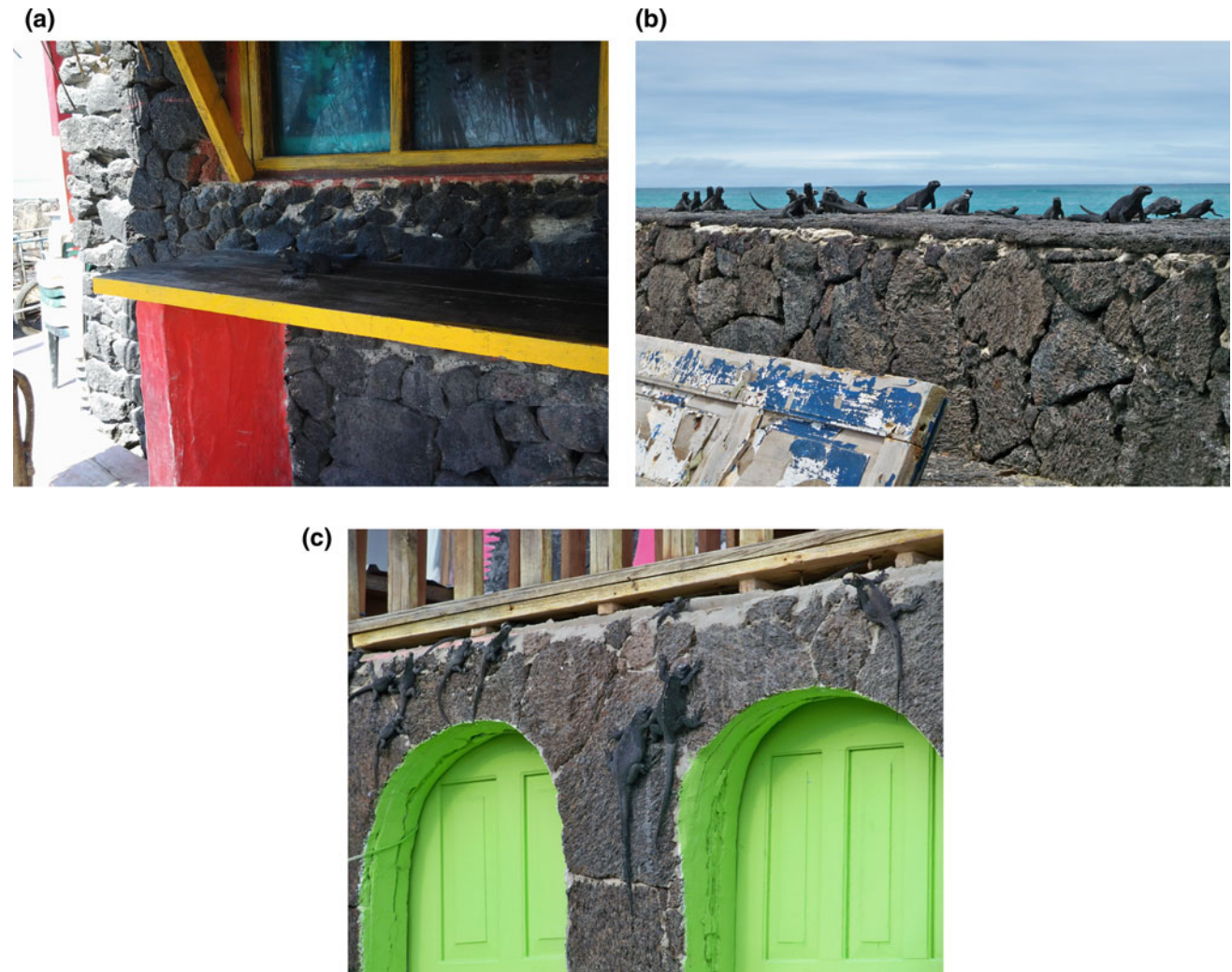
Fig. 2.40 a Basaltic rocks used to cover the exterior walls of a restaurant building in Puerto Villamil. Photo D. F. Kelley b Flat slabs of pahoehoe type lava flow surfaces have been collected and used to
