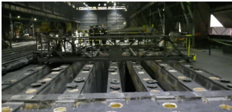
Fig. 6 Test zone in 2018 in Rio Tinto Grande Baie plant
