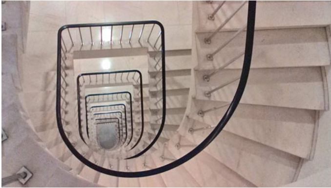
Fig. 16 A spiral staircase consisting of a round part and a square part
