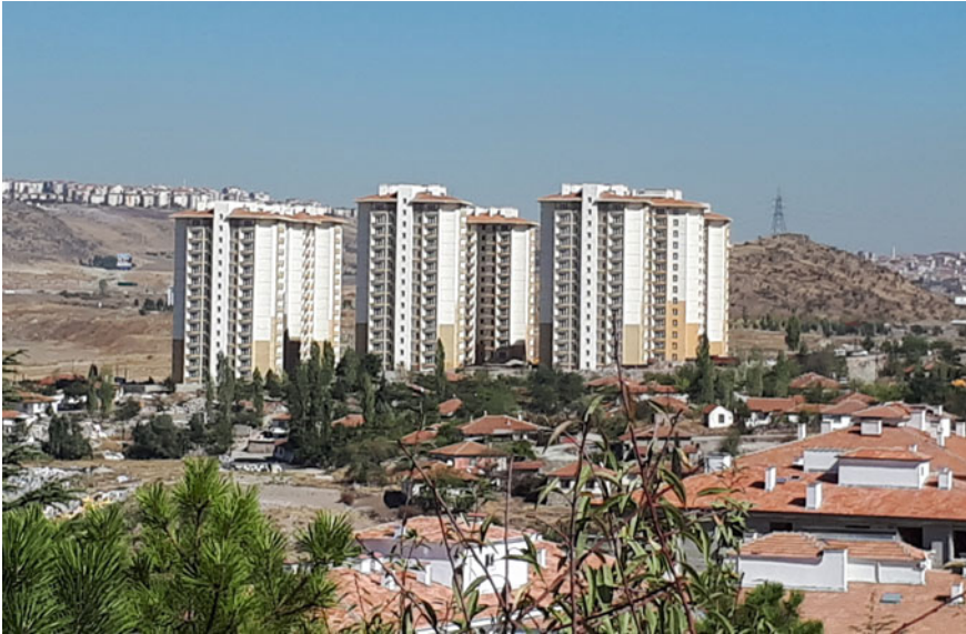
Fig. 8.4 Transformation of squatter housing by HDA. Author's personal archive
