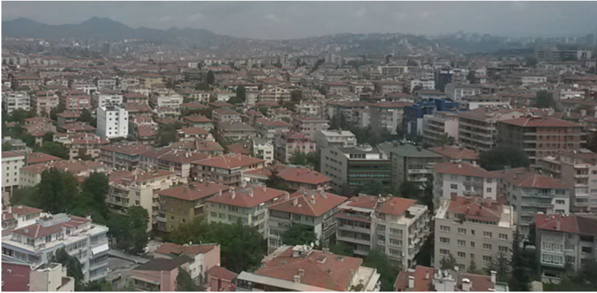
Fig. 8.2 Apartment buildings in planned neighbourhoods. Author's personal archive
