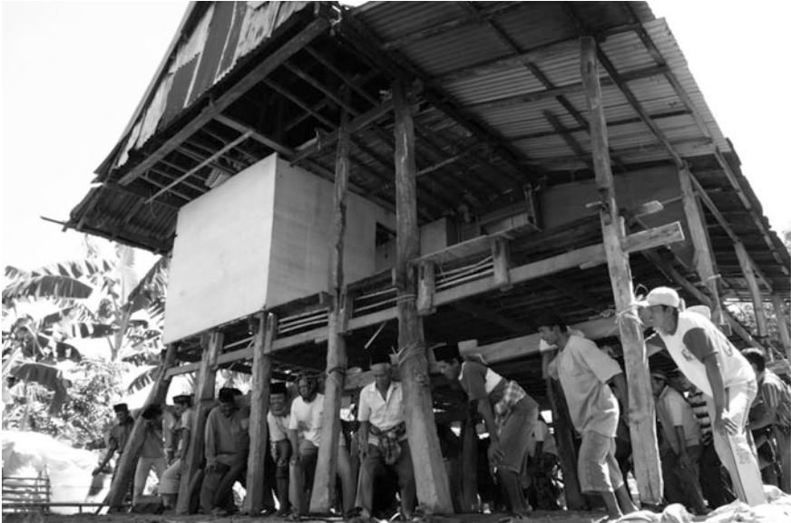
Illustration 14.1 Example of the implementation of gotong royong in moving a house of a neighbouring family in the village. Source Tanoesudibjo (2016)
