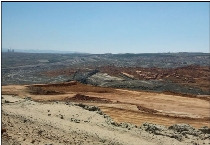
Fig. 11 General view of the June 10, 2017 Amynteon mine landslide
