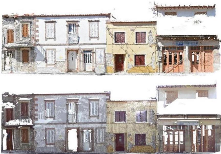
Fig. 7 Point cloud based on terrestrial photogrammetry (up) and laser scanning (down)
