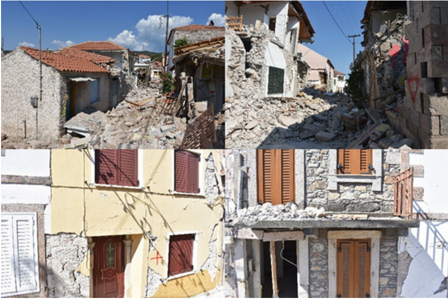
Fig. 4 Street conditions during surveys (up) and two damaged beyond repair buildings of the study area (down)
