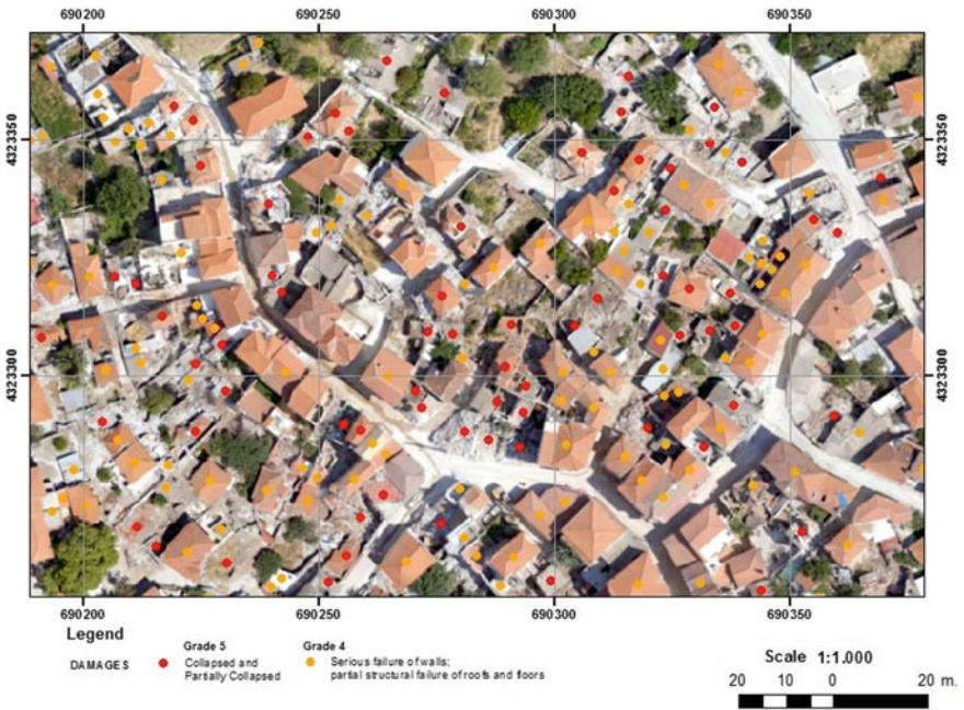
Fig. 11 Orthophoto map of 25th June 2017 at a scale of 1:1.000 showing the NW part of Vrisa settlement which concentrates a large number of building with damages of grades 4 and 5
