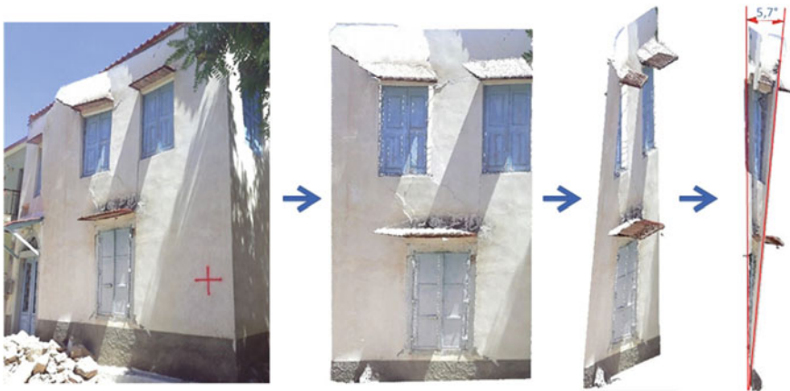
Fig. 13 Measuring the deformation of wall from a TLS point cloud
