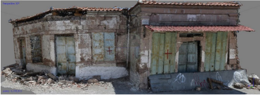
Fig. 12 Part of a 3D model produced by terrestrial photogrammetry
