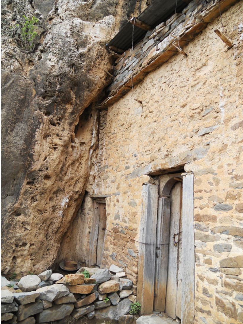
Photo 12.3 Tufa lamination at Ab'aro. A cave in the tufa plug has been enlarged to construct a rock-hewn church. Laminations, steeply dipping to the left and almost parallel to the church wall are clearly visible. Photo Jan Nyssen (2017)
