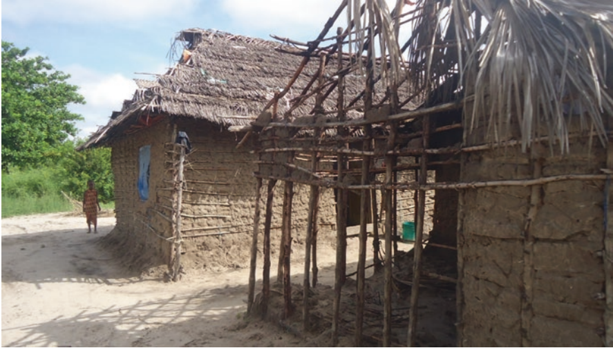
Plate 5 A twig and mud house with makuti (dried palm fronds) thatched roof in Mchungu village. While such houses are widespread in Mchungu, in Nyamisati, they are commonly seen in the periphery of the village indicating that poverty was much more widely spread in Mchungu than in the latter village. (Source: Photo by Anselm Mwajombe, May 2016)
