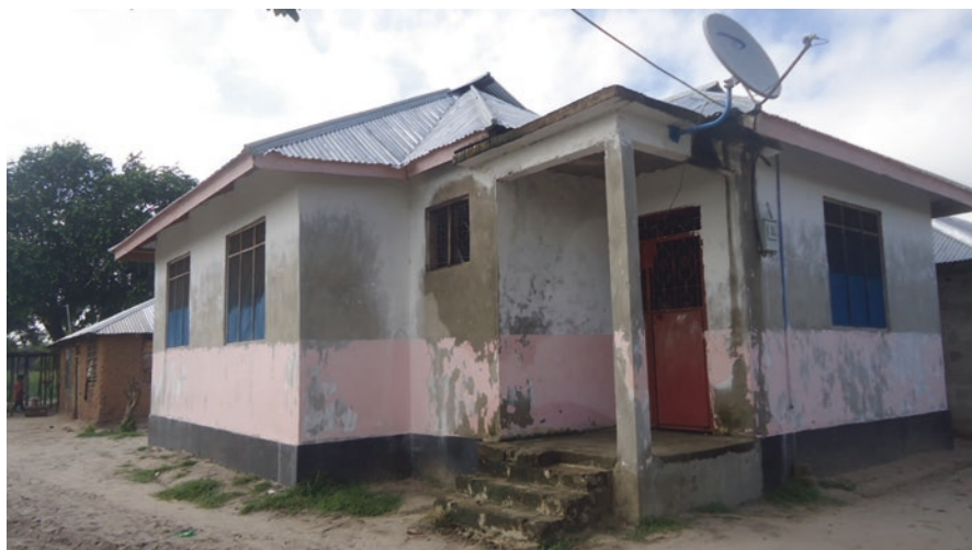
Plate 3 An iron-roofed brick house for a ‘well-off’ household in Nyamisati village. Note the TV dish on the roof. (Source: Photo by Anselm Mwajombe, May 2016)
