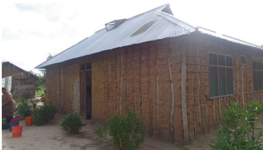
Plate 4 A hard wood mud house with corrugated iron roof OF 'middle wealth group' in Nyamisati village. (Source: Photo by Anselm Mwajombe, May 2016)
