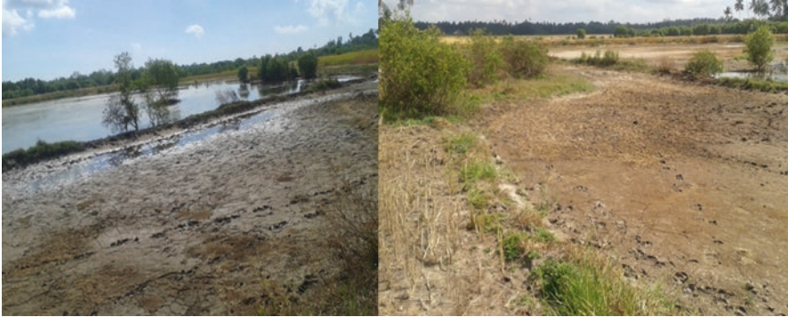
Plate 2 Professionally made ridges at Wingwi which were built by the help of the central government to protect rice farms from coastal flooding. (Source: Photos by the Authors, 2015)
