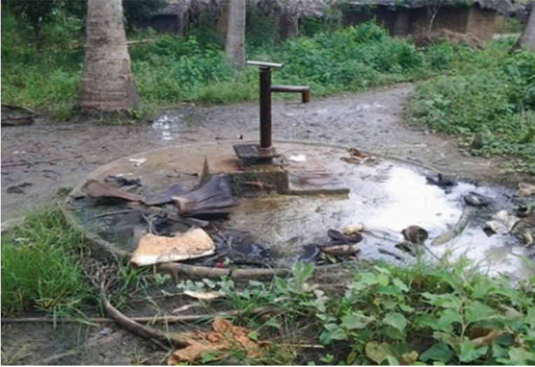
Plate 3 Abandoned borehole due to increase of salinity in Msaraza village
