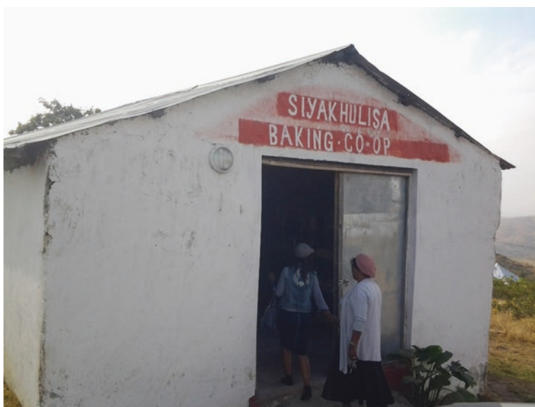
Fig. 13.11 Cooperative bakery in Eastern Cape (Qandu)
