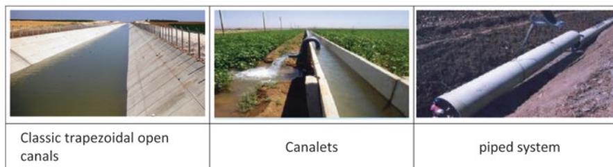
Fig. 7.3 Typical open canal, canalet, and piped systems used in Turkey’s irrigation schemes (DSI 2017)
