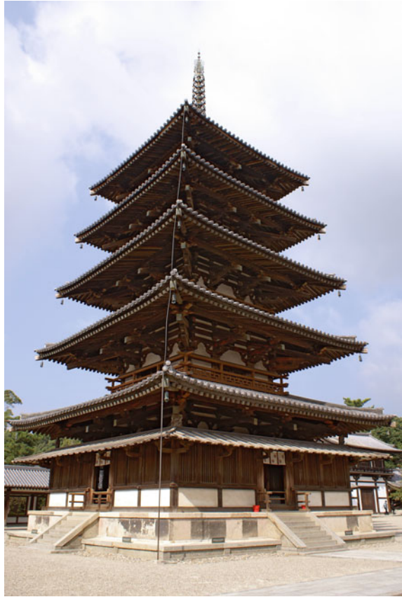
Fig. 4 Hōryū-ji in Japan, is one of the oldest wooden buildings in the world
