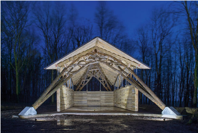
Fig. 4 AA, Woodchip Barn, Architectural Association: pavilion robotically fabricated and made by natural and low-engineered wood. © AA, Architectural Association, Valerie Bennett
