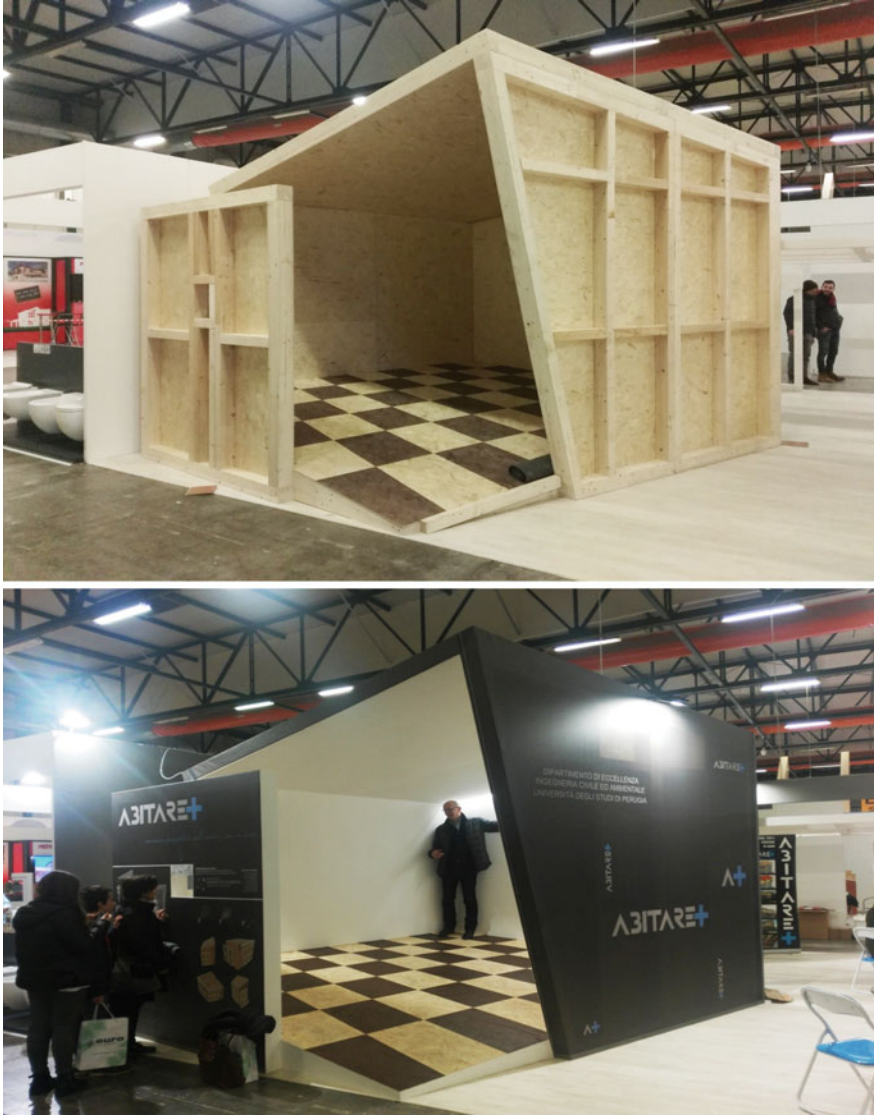
Fig. 31 The installation of the Ames' room: the timber structure and the final realization
