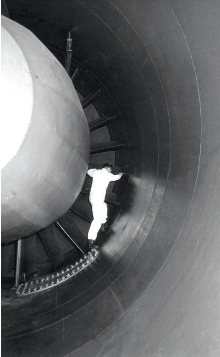
←↑The HST of the NLL was – and is – impressive, both from the outside (see § 3.2.1) and from the inside. Its operation demanded a large increase of the output of the power plant of the institute. The operators and researchers of the tunnel were located in a special room. By 1960 one of the means to get control of the operation of the tunnel was the use of closed-circuit television. (courtesy of Stichting Behoud Erfgoed NLR)
