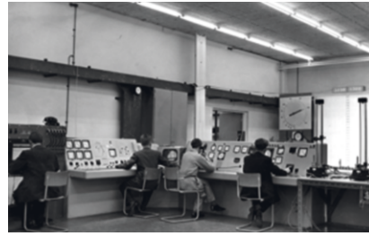
←↑The HST of the NLL was – and is – impressive, both from the outside (see § 3.2.1) and from the inside. Its operation demanded a large increase of the output of the power plant of the institute. The operators and researchers of the tunnel were located in a special room. By 1960 one of the means to get control of the operation of the tunnel was the use of closed-circuit television. (courtesy of Stichting Behoud Erfgoed NLR)
