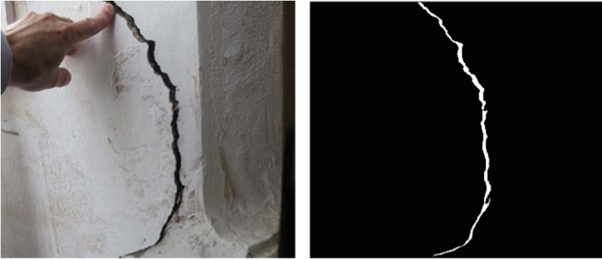
Fig. 4. Automatic crack detection in a concrete column. Left image is the input crack image, right image is the detected binary crack map
