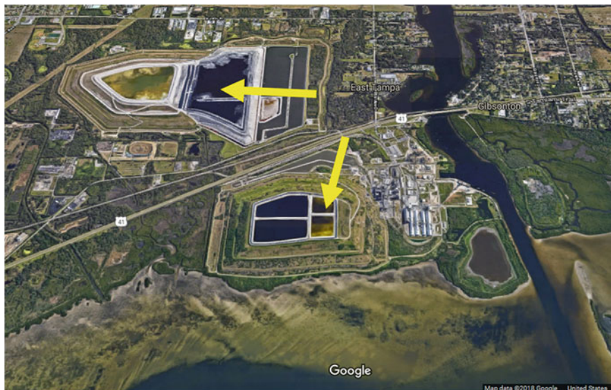
Fig. 5.18 Two gypsum stacks (indicated by yellow arrows) situated adjacent to Tampa Bay and the Alafia River. (Google Maps)
