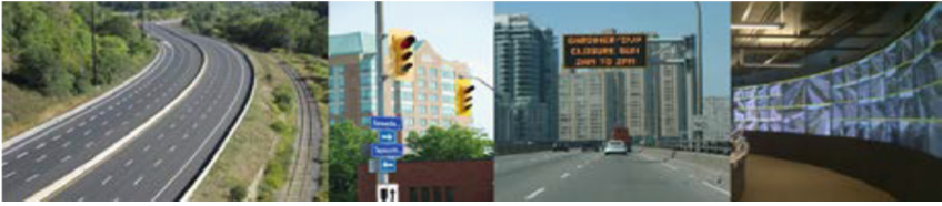
Fig. 6. Roads with VMS systems [6].
