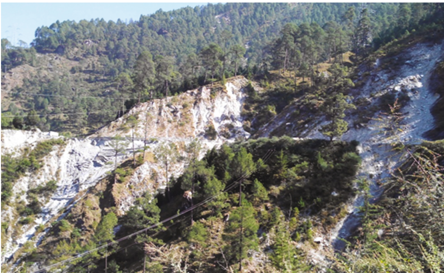
Fig. 2. A panoramic view of the landslide
