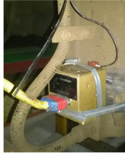
Fig. 1. Bogie mounted gyrometer and accelerometer
