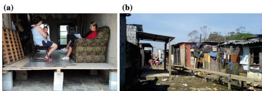
Fig. 14.4 Social assistance (a) and the situation of the illegal houses on the floodplains of the Tietê River (b). Photos: Schutzer, 2017
