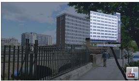
Fig. 16. The Metropolitan hotel before alignment.
