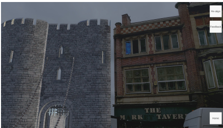
Fig. 21. Over time, with continuous changes in orientation, calculation drift can occur, producing a slight misalignment between the virtual model and the real world, which affects the depth masking process.
