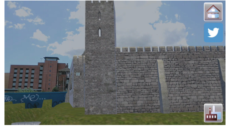
Fig. 20. A view of the castle from the north side taken shortly after midday. The sun is high in the sky. The front face of the buttress supporting the wall is brighter than in Fig. 19, as are the angled upper surfaces of the crenellated battlements.
