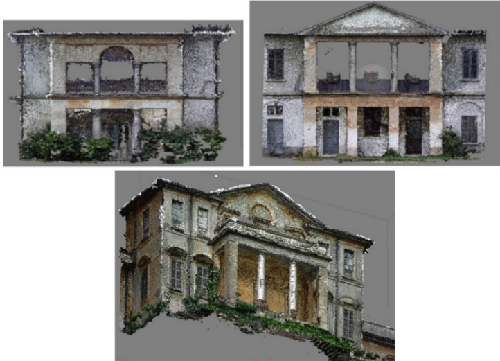
Fig. 2. DP dense clouds of Cascina Casalta (top) and Villa Mirabellino (down). The first includes three loggias directed to different axis in the landscape. Villa Mirabellino, on a hill is the end point of a green perspective axis from Villa Mirabello (Color figure online)
