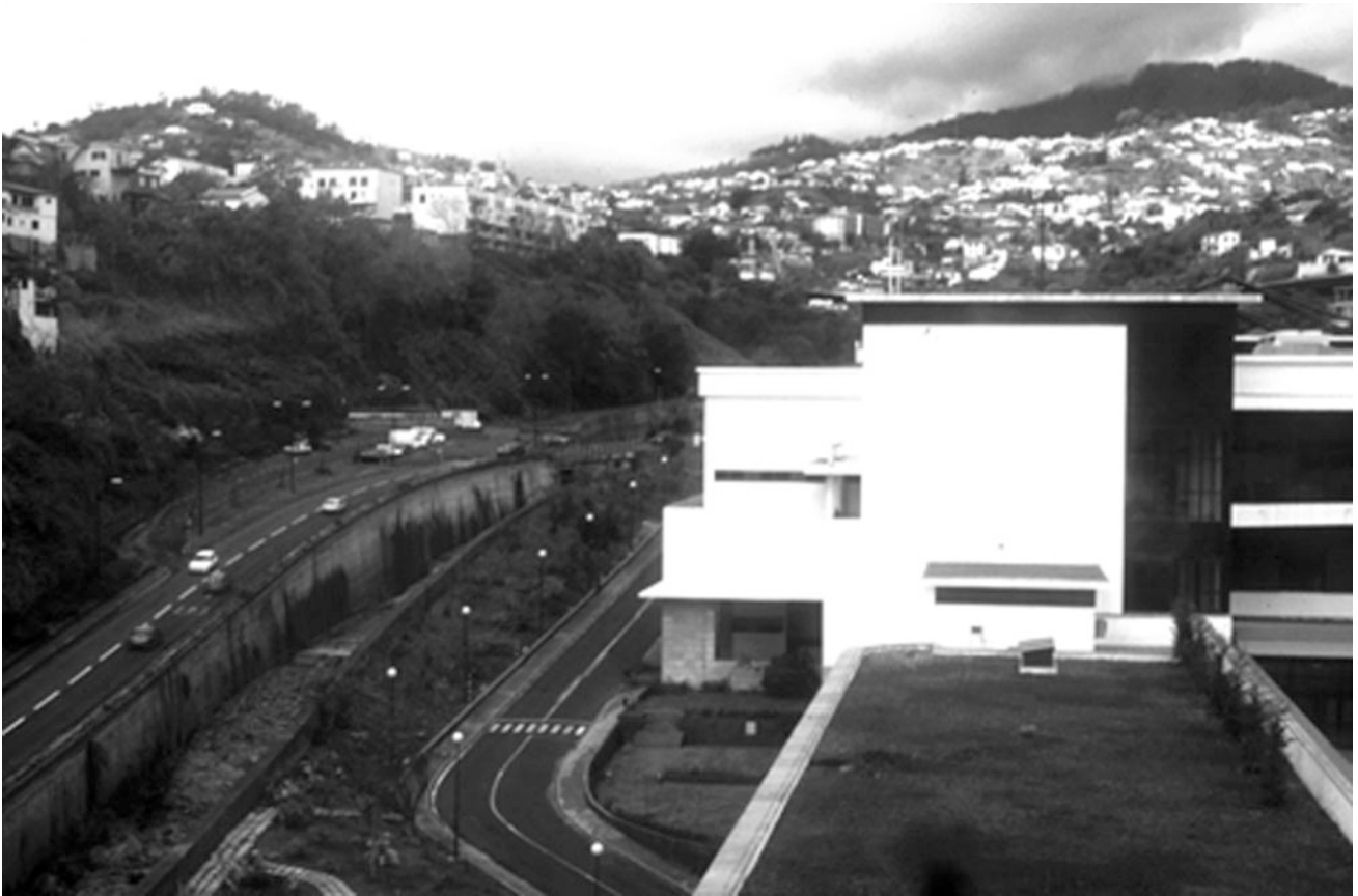
Fig. 2 Example of changes in the fluvial morphology by narrowing the original riverbeds, and reducing the original section of the “Ribeira de Santa Luzia” river within Funchal city
