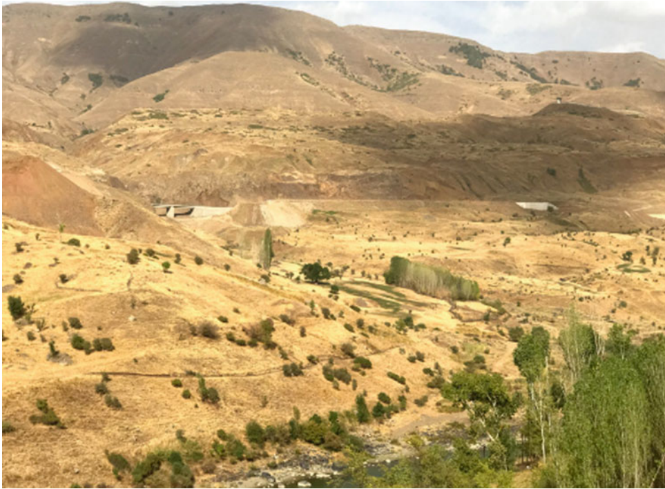
Fig. 3 A general view of a large landslide in the study area (typical hummocks are seen clearly)
