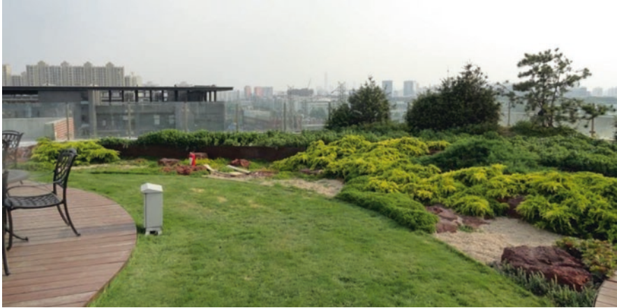
Fig. 7 A showpiece green roof in Beijing (May 2017)
