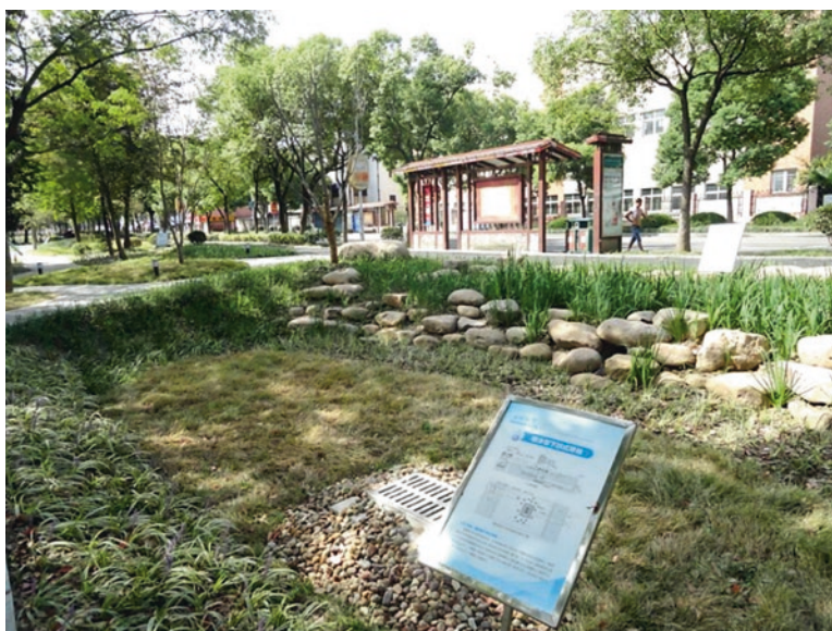
Fig. 6 Sponge City component "Sunken Greenbelt" in Jiaxing (September 2016)
