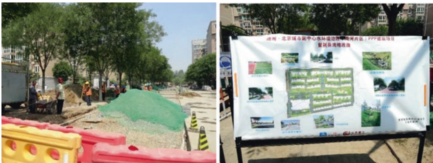
Fig. 8 Sponge City construction site in Tongzhou District, Beijing (May 2017)
