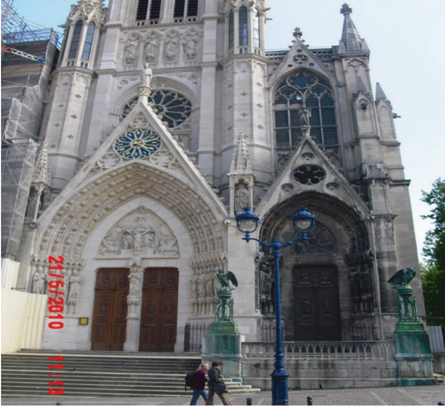
Fig. 2.1 Cleaning of a church facade
