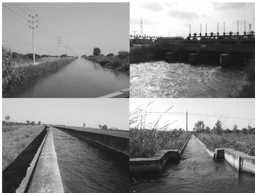
Fig. 15.3 Irrigation facilities in the Lower Seyhan Irrigation Project (Top left: Conveyance canal; Top right: Diversion weir; Bottom left: Secondary canal; Bottom right: Tertiary canal). Source Photos by Chieko Umetsu
