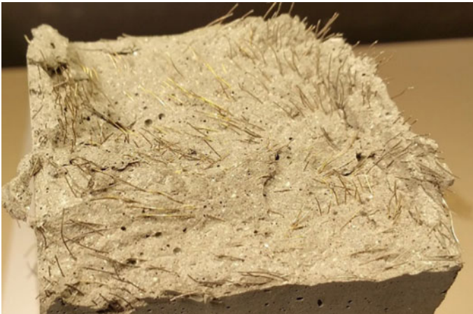
Fig. 4 Cross section of the collapsed specimen PK05Wb
