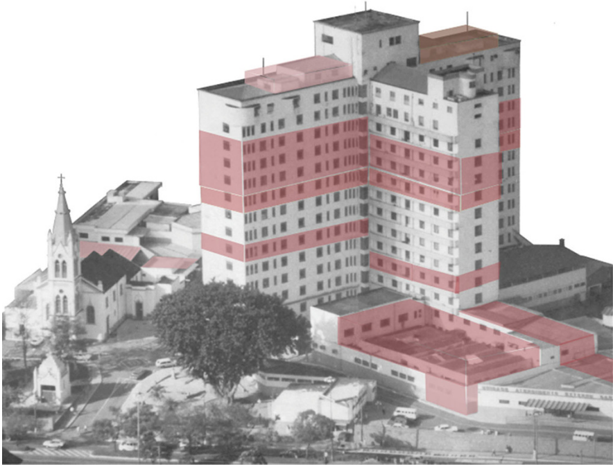
Fig. 15 Juiz de Fora's Holy House of Mercy, Refurbishments until 2017. Source: Author's own illustration (2017)
